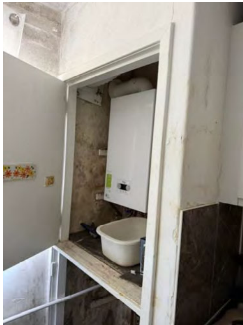
Photograph 3: Kitchen: boiler and cupboard (no carbon monoxide detector). As 4 November 2025.
