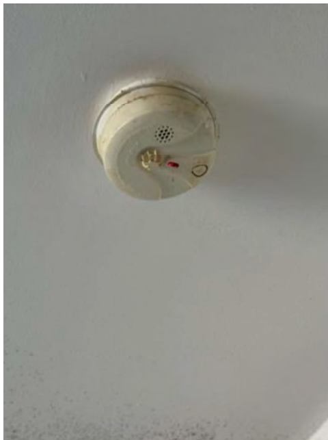
Photograph 5: Kitchen: Old heat detector – not working – red light illuminated
