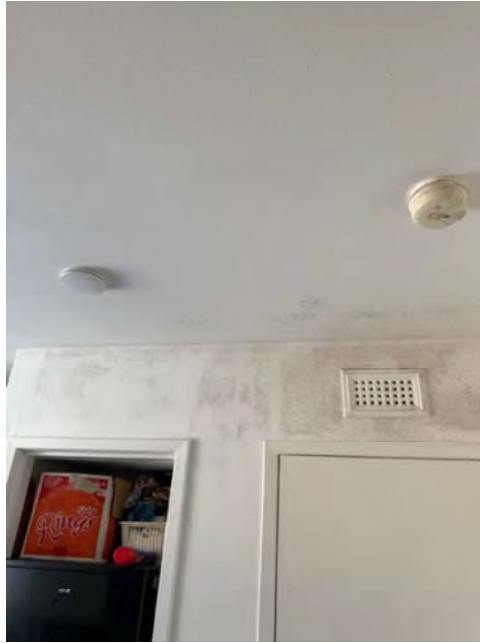
Photograph 5: Kitchen: Old heat detector – not working – red light illuminated
