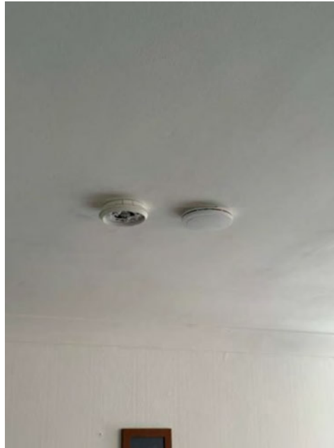
Photograph 7: Living room: carbon monoxide detector above fireplace. As November 2025.
