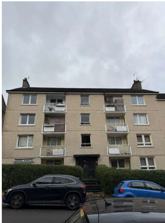
Photograph 1 (taken on 4 November 2025): front elevation. The subject property is top right in the block.
