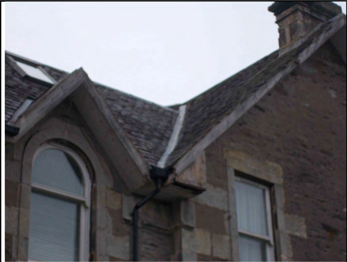
16. Valley Gutter over stair to Attic Level.
