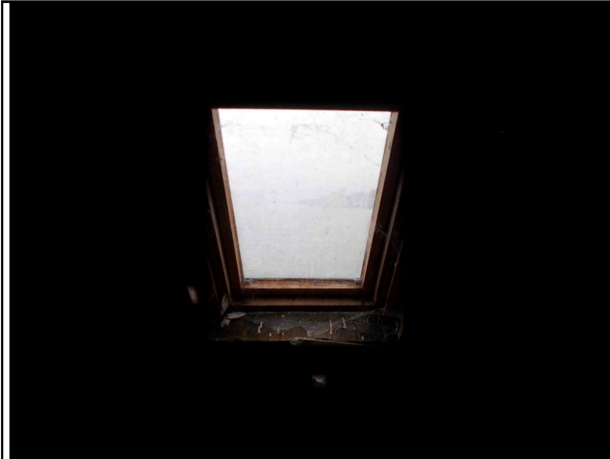
15. Velux window above Living Room below.
