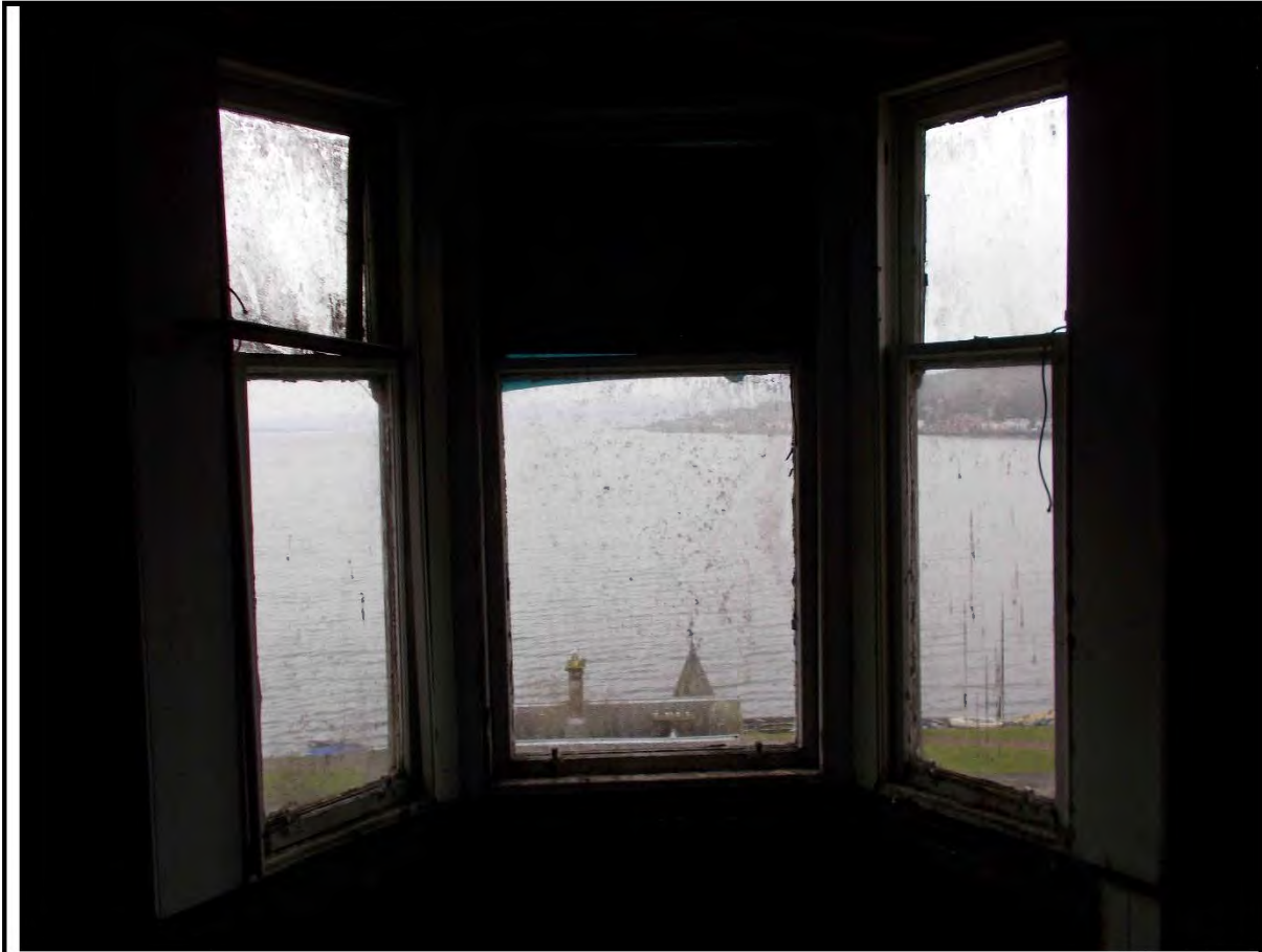
12. Attic Level Bay Window in poor condition.
