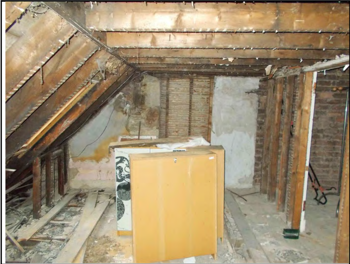
11. Stripped out attic area.
