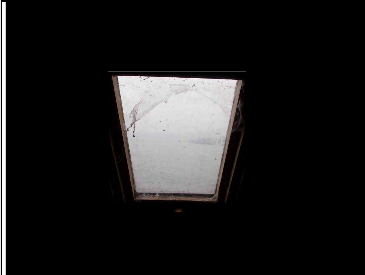
13. Velux window over Dressing Room below.
