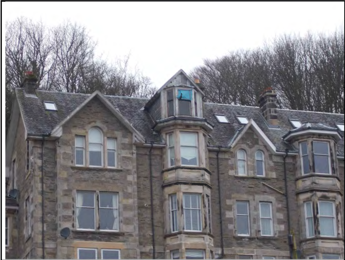
18. Detail of Attic Level Bay Window
