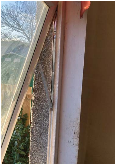
Living room window 12 December 2025 New fitted hinge has been installed.
