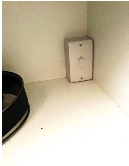
Enclosed cooker control unit recently fitted and located in kitchen
