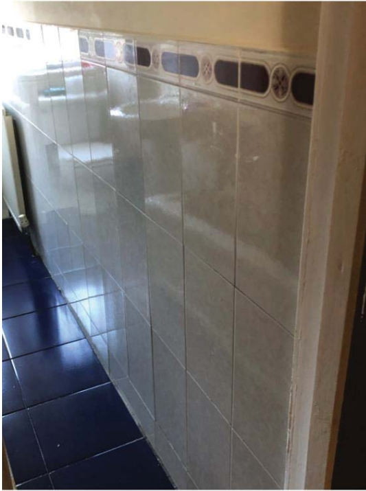
Photo 6 – Bathroom tiling reinstated throughout
