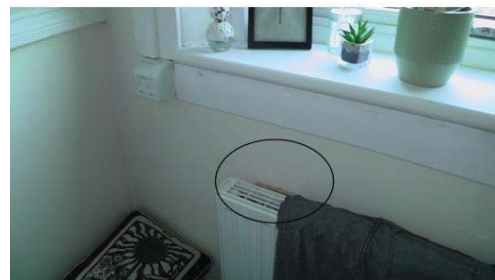
Photo 9 – Radiator now secured to wall
