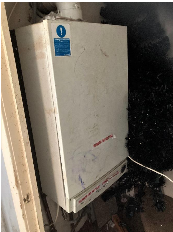
4. Wall mounted gas boiler
