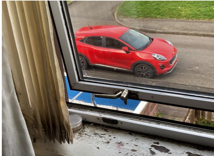
13. Condensation at front bedroom window
