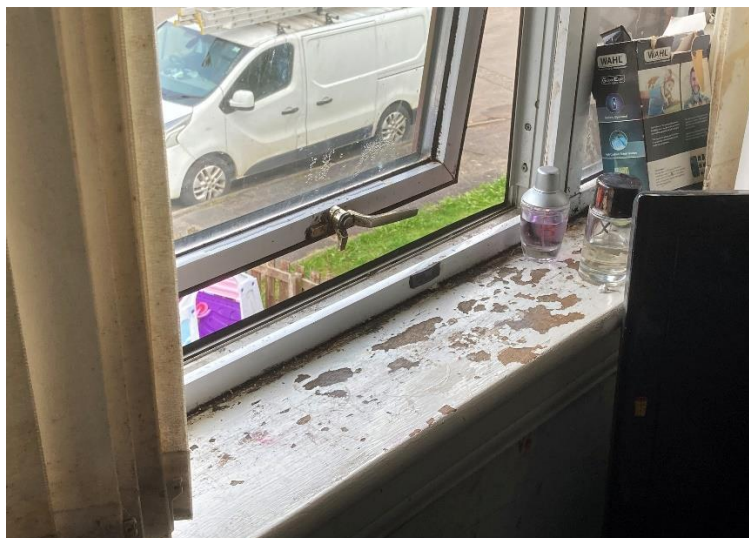
12. Condensation at front bedroom window
