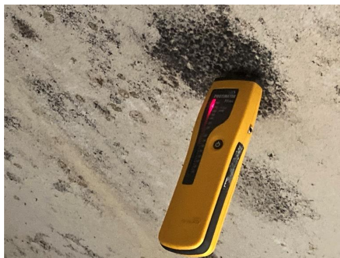
9. Damp "ceiling plaster" in attic
