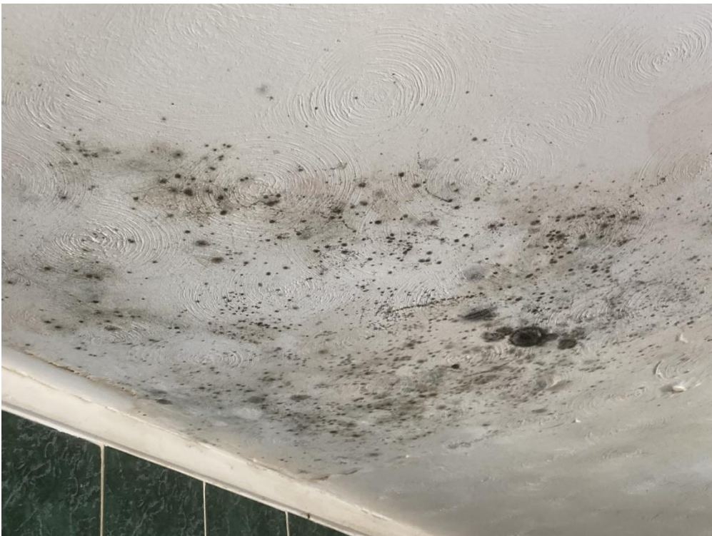
27. Damp staining kitchen ceiling below bathroom
