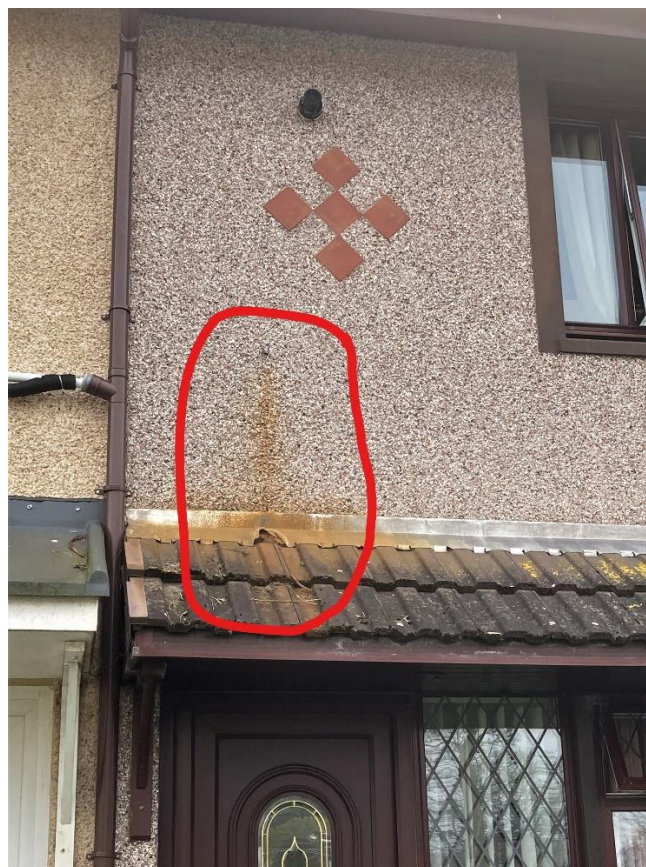
29 Residual staining below overflow pipe from boiler
