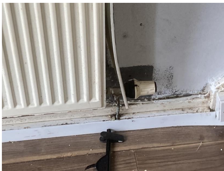
21. Broken radiator panel and condensation staining in hall
