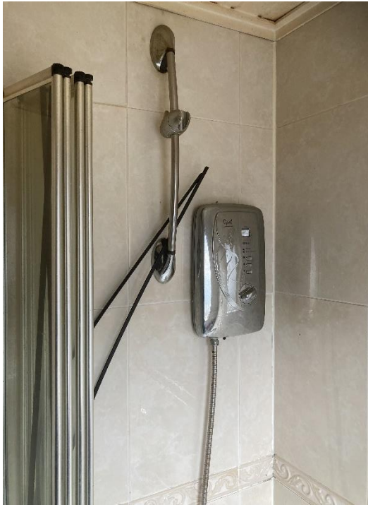
Broken electric shower and shower head attachment
