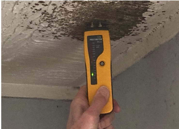
10. Staining (dry) front bedroom ceiling
