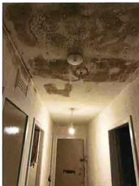
Photograph 2: Hallway: Smoke detectors – newly installed and old. Indicates presence of mould to ceiling
