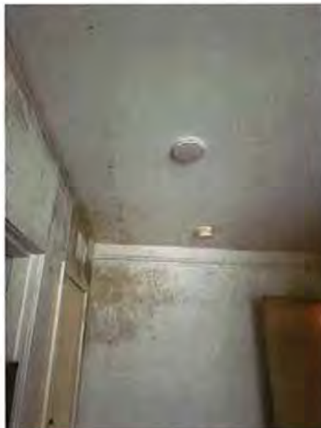
Photograph 5: Kitchen: newly installed smoke detector and old heat detector (not interlinked). Indicates presence of mould
