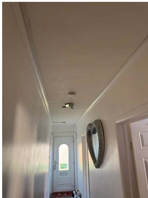
Photograph 7: Hallway: smoke detector
