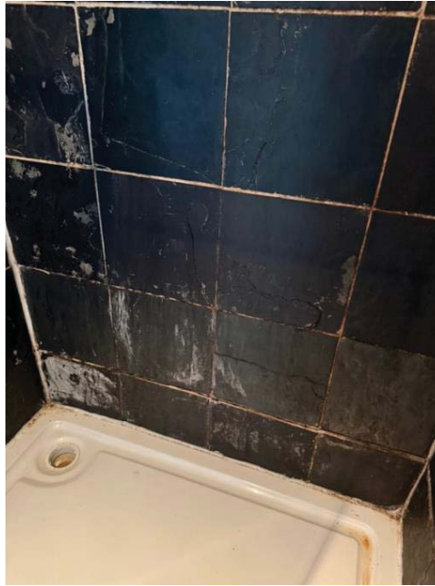
Photograph 18: Bathroom: Shower tray and tiles to walls in poor condition
