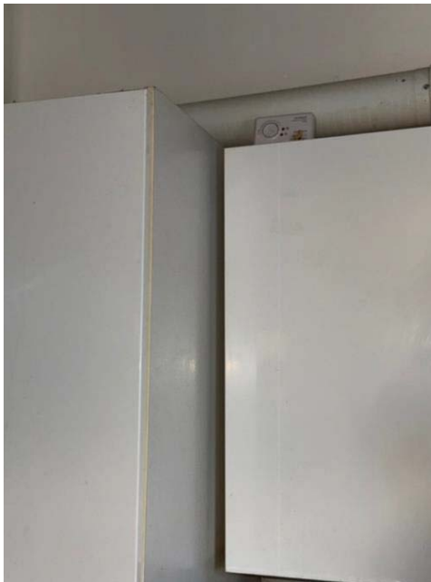
Photograph 11: Kitchen: Carbon monoxide detector
