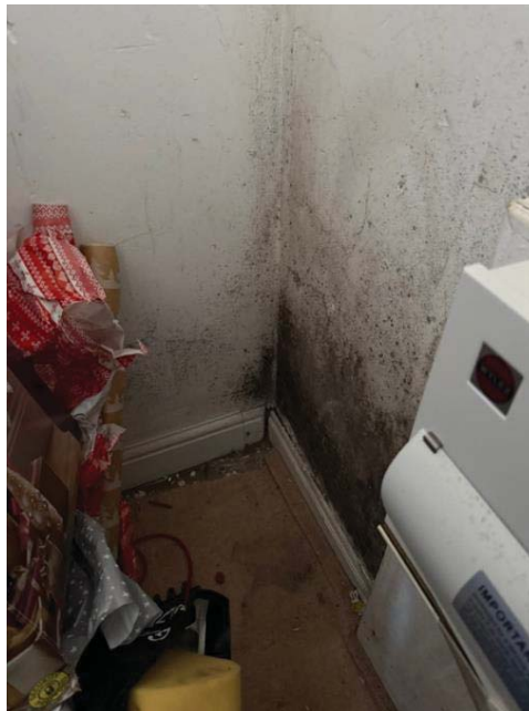
Photograph 15: Hall cupboard: mould to walls
