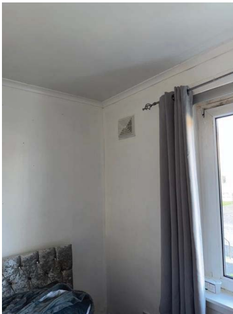
Photograph 5: Bed 1: vent to external wall
