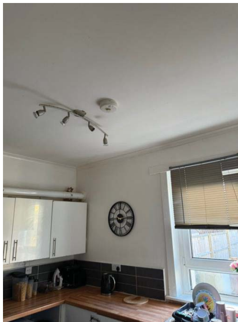
Photograph 9: Kitchen: heat detector
