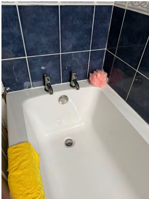
Photograph 7: Bathroom: bath with new sealant
