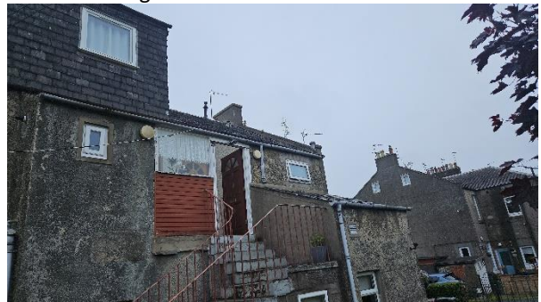
12 Rear Elevation of property.
