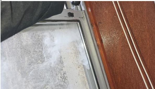
7 Smoke testing – escape evident.
