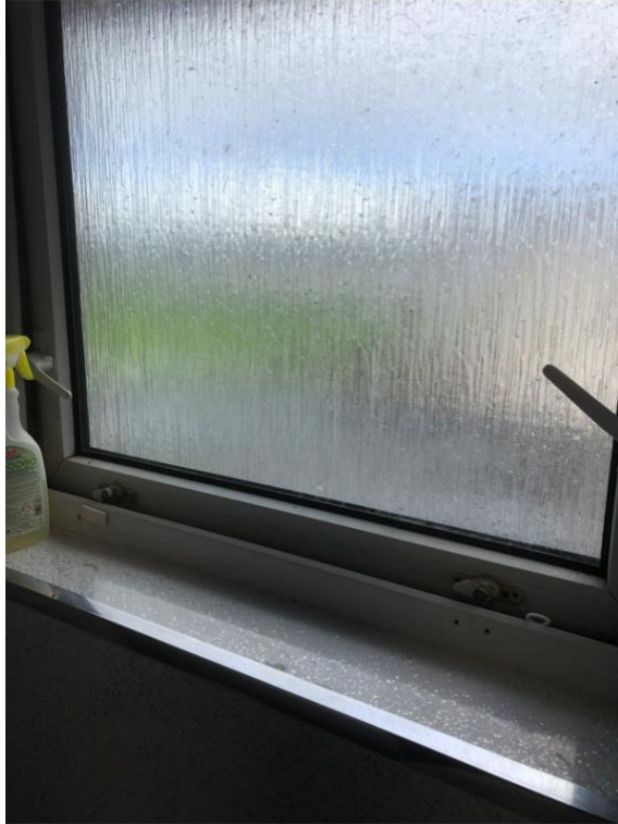
Photo 6 – Life-expired Bathroom window
