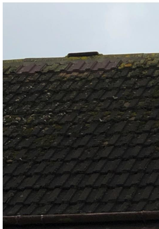
Photo 9 – Recent roof repair
