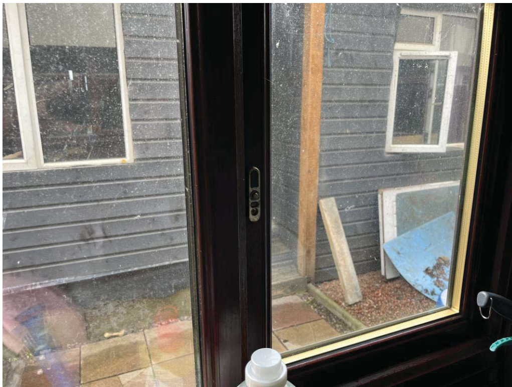
Missing/broken handles on the kitchen windows
