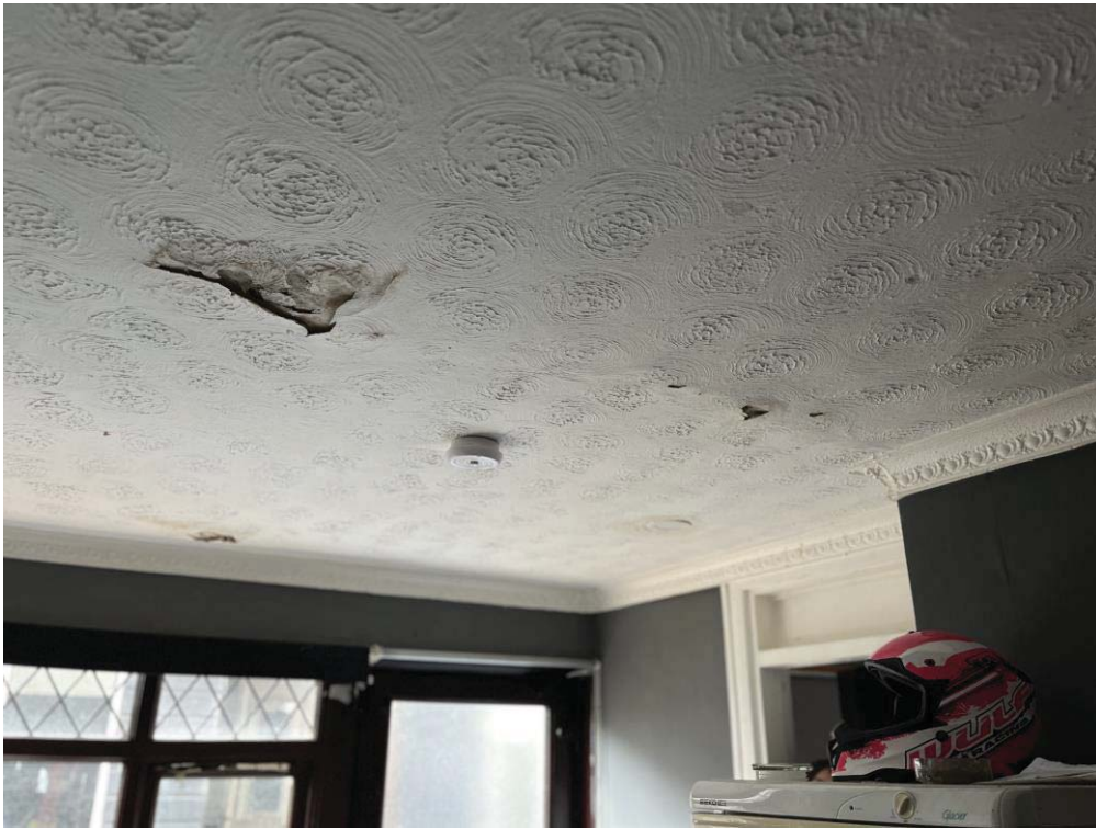
Multiple stains and signs of water damage on the kitchen ceiling
