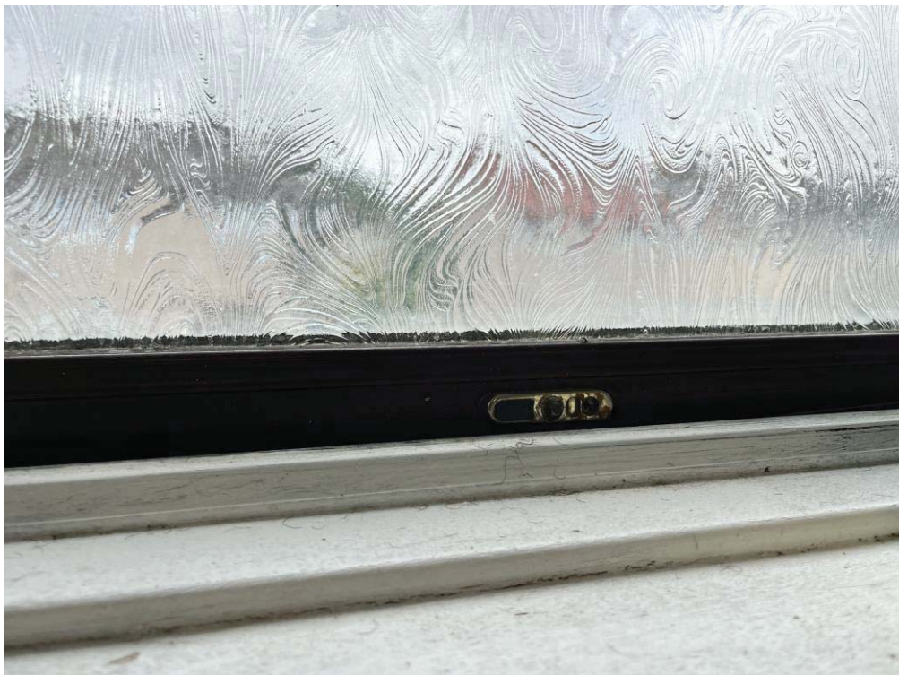
Missing/broken handle on the bathroom window
