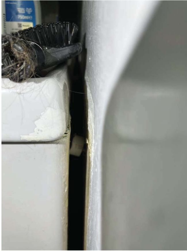
Gap between the toilet cistern and the wall in the ground floor toilet
