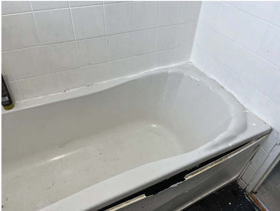
Damaged and loose bath panel and defective surrounds to the bath
