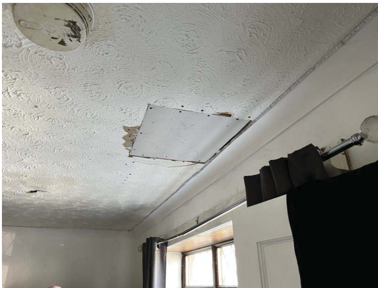
Damaged and bowed ceiling in the living-room
