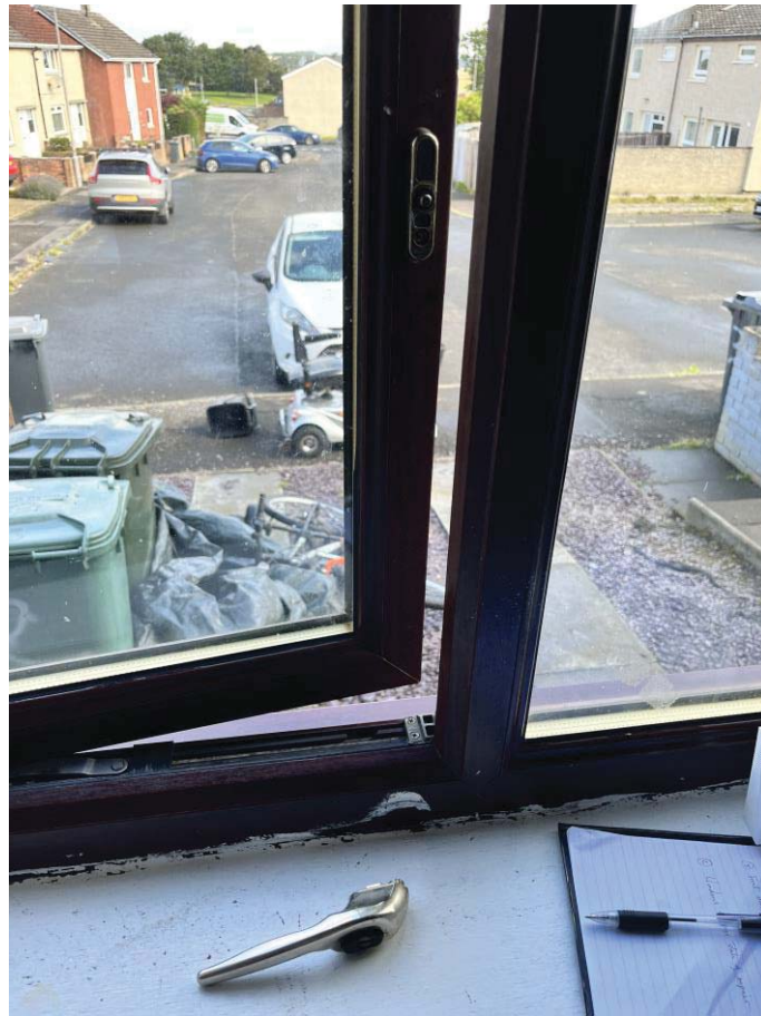
Broken window handle in the living-room
