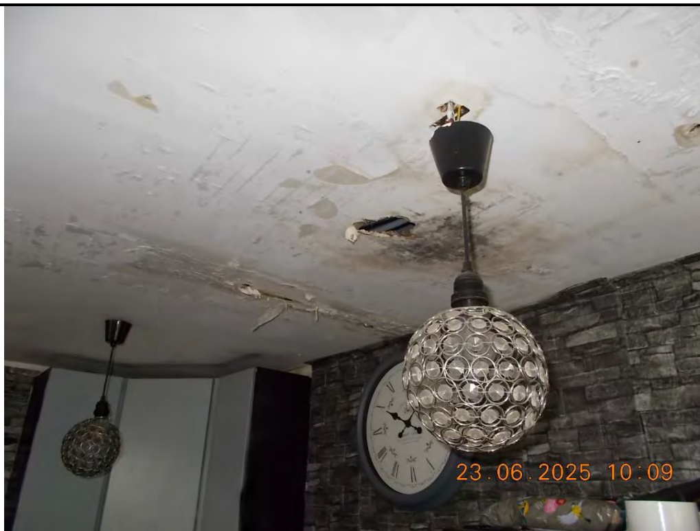
18. Mould on ceiling in Kitchen
