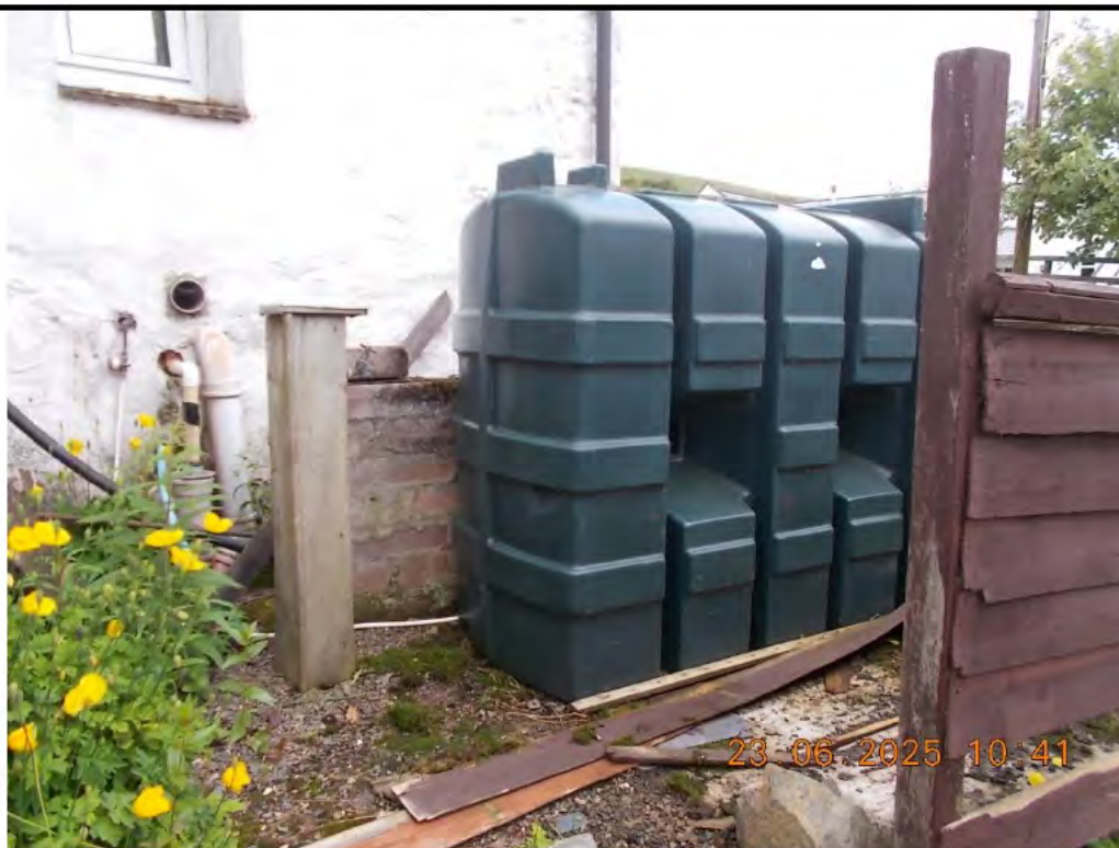
13. External oil storage tank
