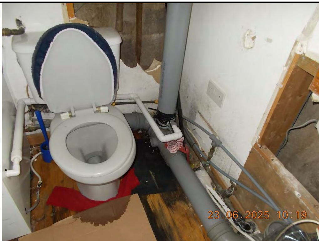
28. Leaking pipes in Downstairs WC
