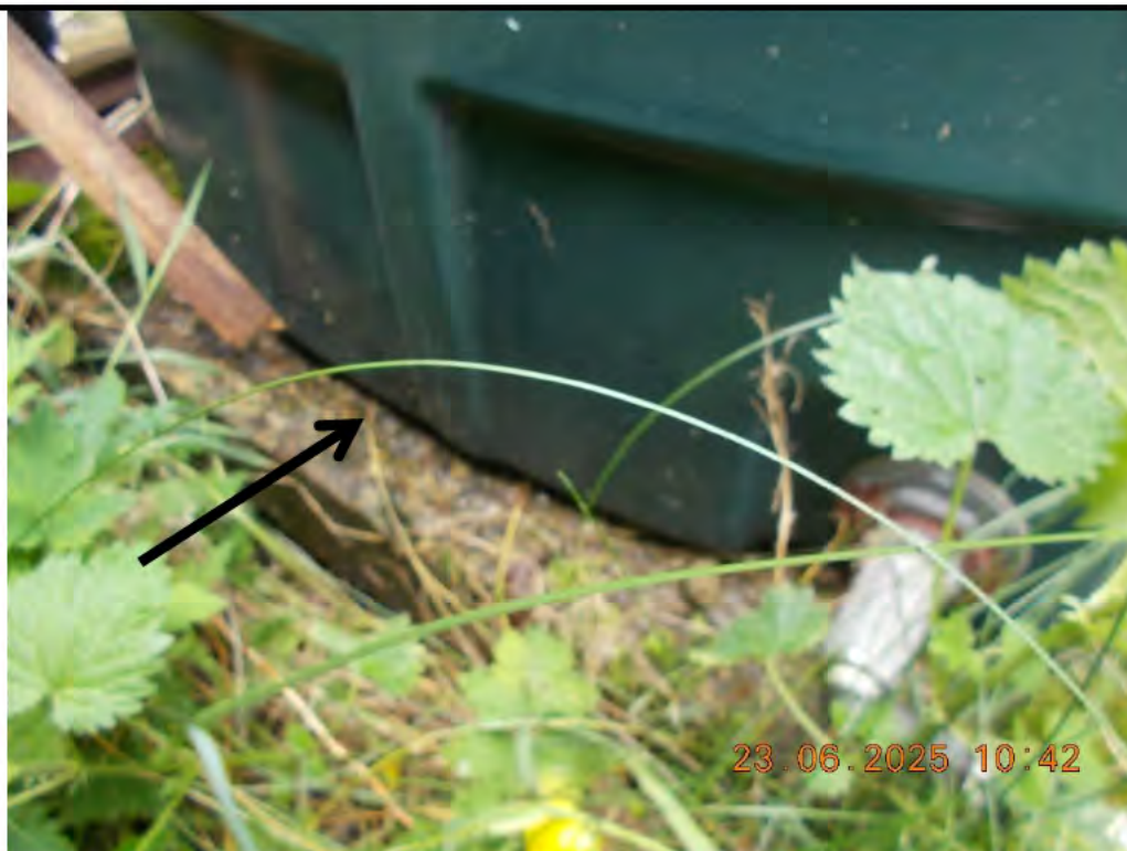
14. Oil leak from tank (arrow added)
