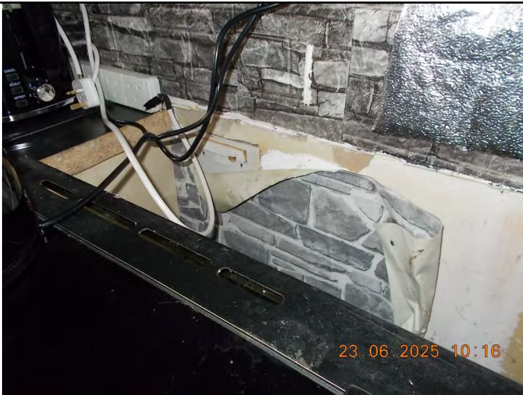
4. Socket outlet on wall behind cooker
