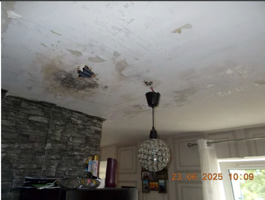
1. Kitchen ceiling light fitting also holes and mould growth
