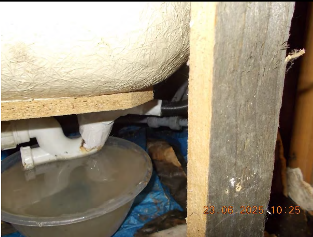
30. Leaking pipes in Bathroom
