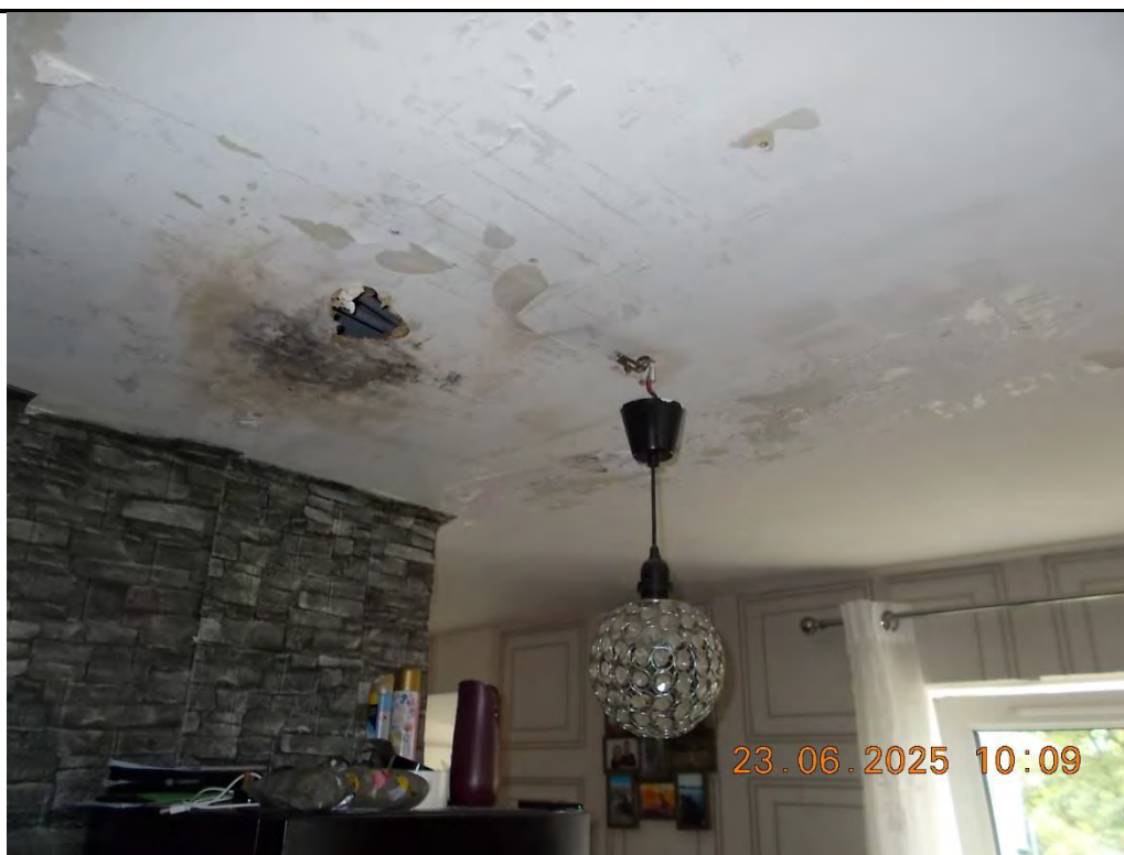
17. Mould on ceiling in Kitchen
