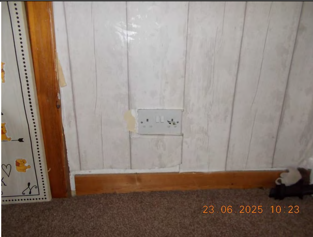
9. Damaged socket outlet in upper hallway
