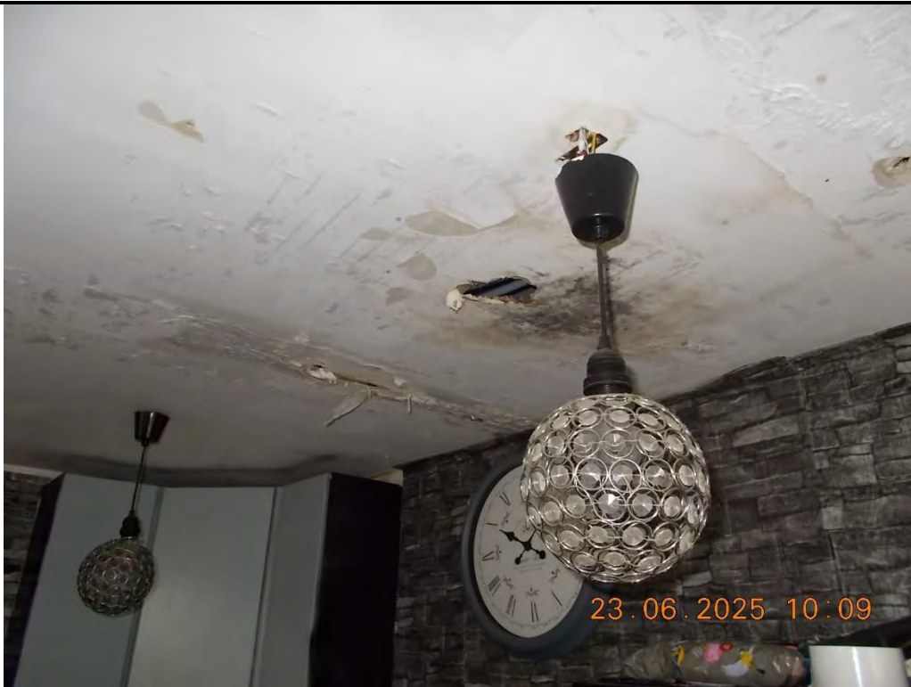
2. Kitchen ceiling light fitting also holes and mould growth
