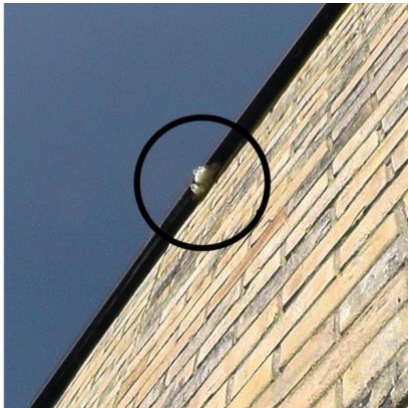
Photo 4 – Insulation blown out from roof space
