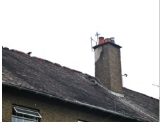
External - front elevation - render to second chimney head patched
