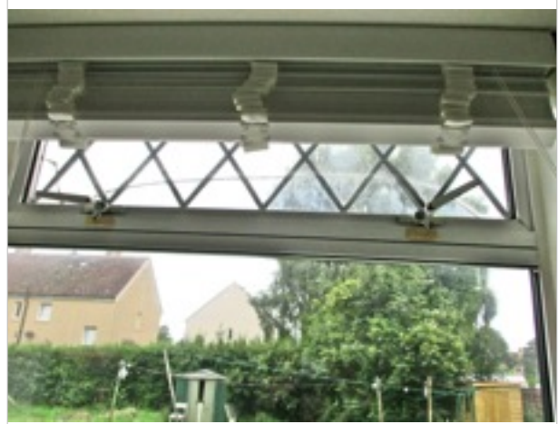
Kitchen - top hung section of glazing cracked
