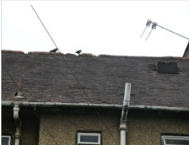
External - rear elevation - several damaged/missing roof and ridge tiles and broken sections of gutter
