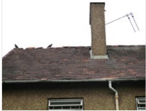
External - front elevation - several damaged/ missing roof and ridge tiles
