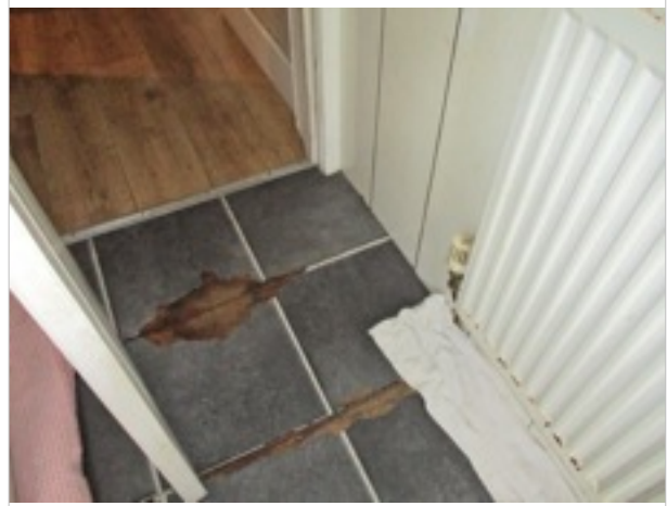
Bathroom - flooring damaged adjacent to radiator
