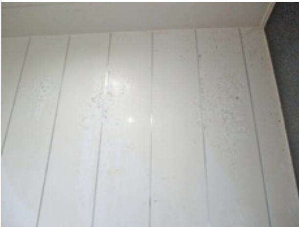
Bathroom - widespread black spot mould to wall cladding
