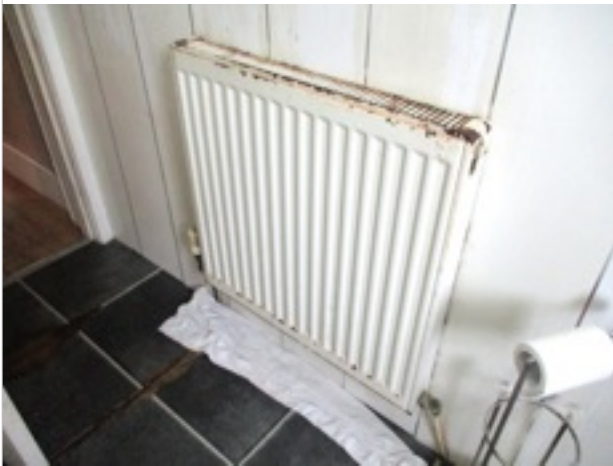
Bathroom - wall mounted radiator - extensive corrosion
