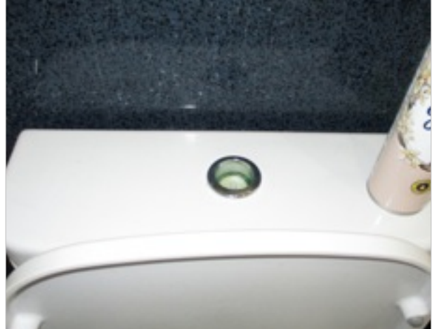
Bathroom - toilet flush button missing
