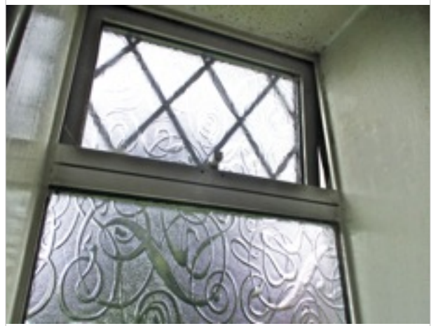
Bathroom - window handle broken
