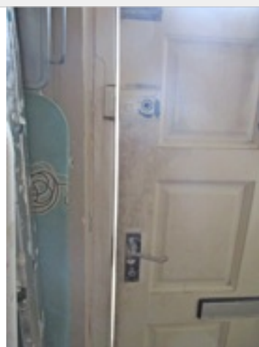
Hall - full height gap to left side of front door
