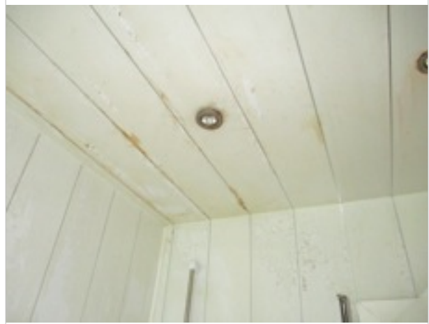
Bathroom - widespread black spot mould to wall and ceiling cladding
