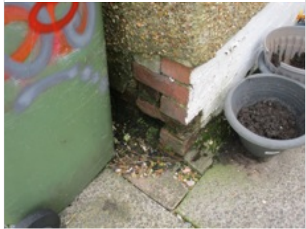
External - area of spalling render/exposed damaged base bricks at corner of rear elevation and gable wall
