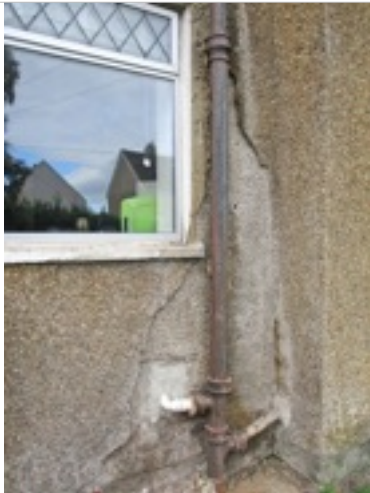
External - rear elevation - extensive damage/ spalling to render surrounding cast iron waste pipe
