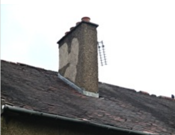
External - front elevation - render to chimney head patched
