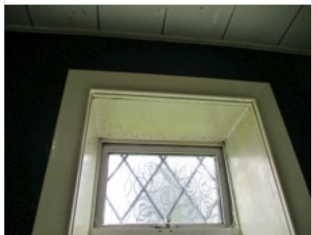
Bathroom - black spot mould to window surround
