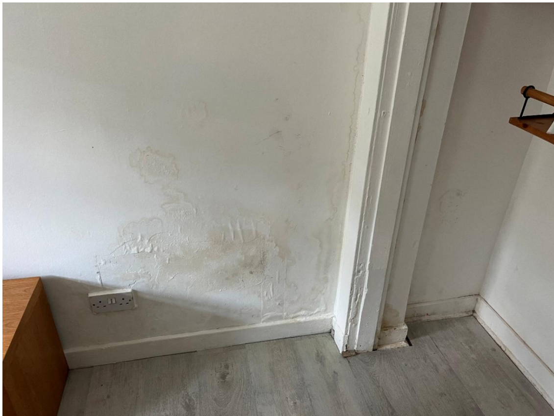
Damp staining on gable wall of second Bedroom.
