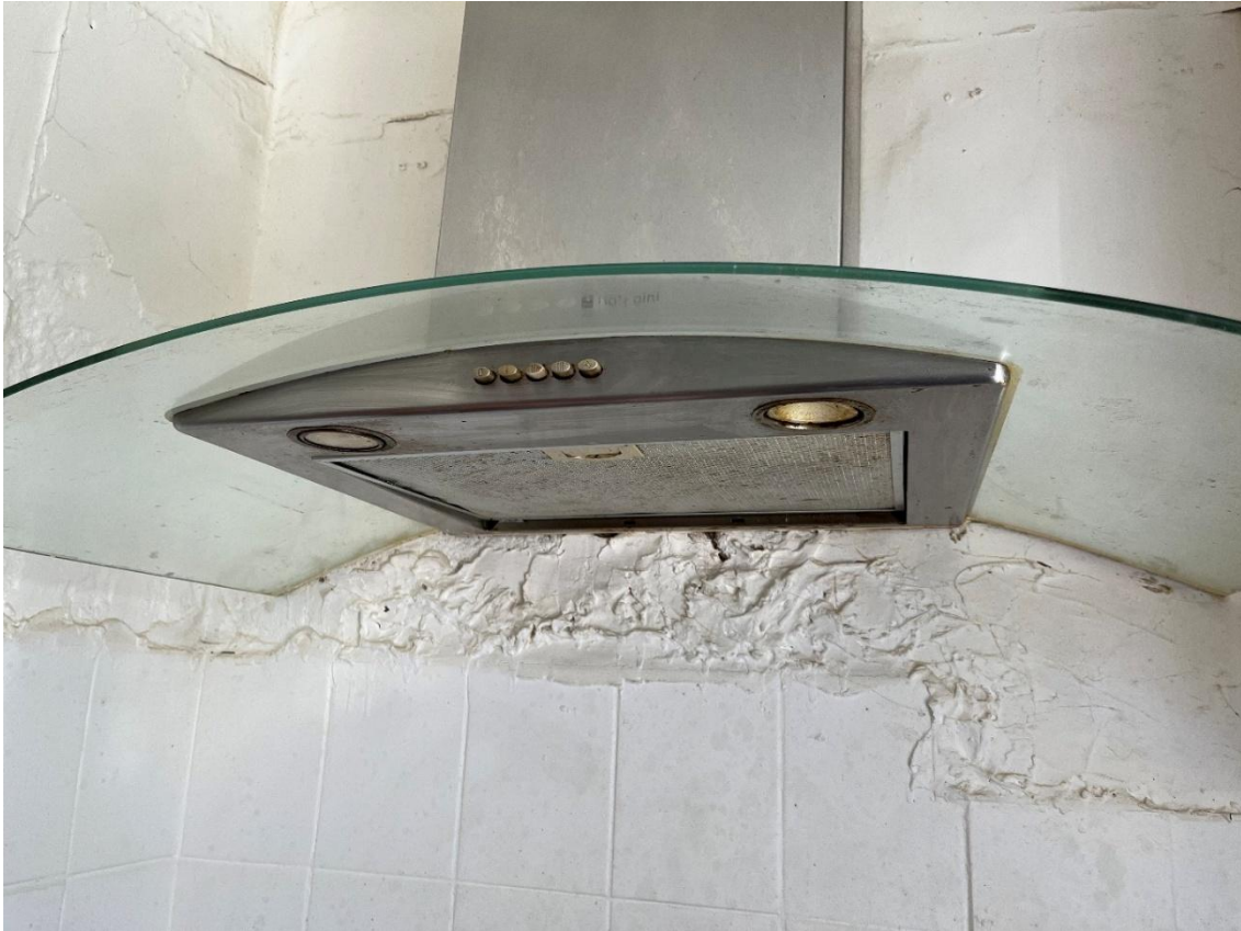
Cooker hood showing defective lights and loose/damaged filter.
