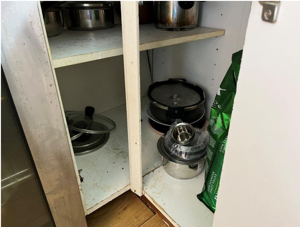
Kitchen cupboard showing missing door, missing base trim and damaged rear panel.
