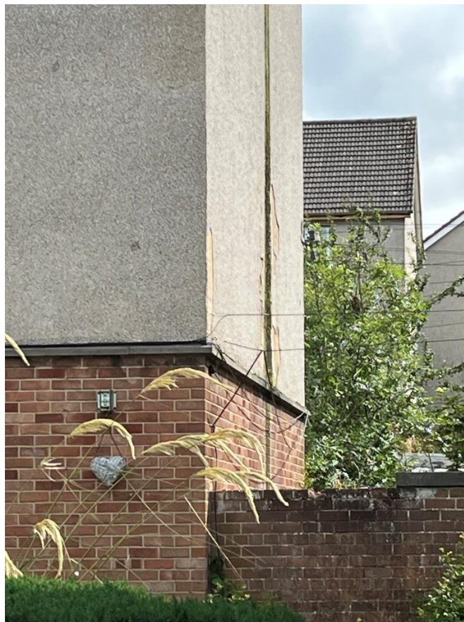
Water running from overflow pipe of second floor flat above subject property.
