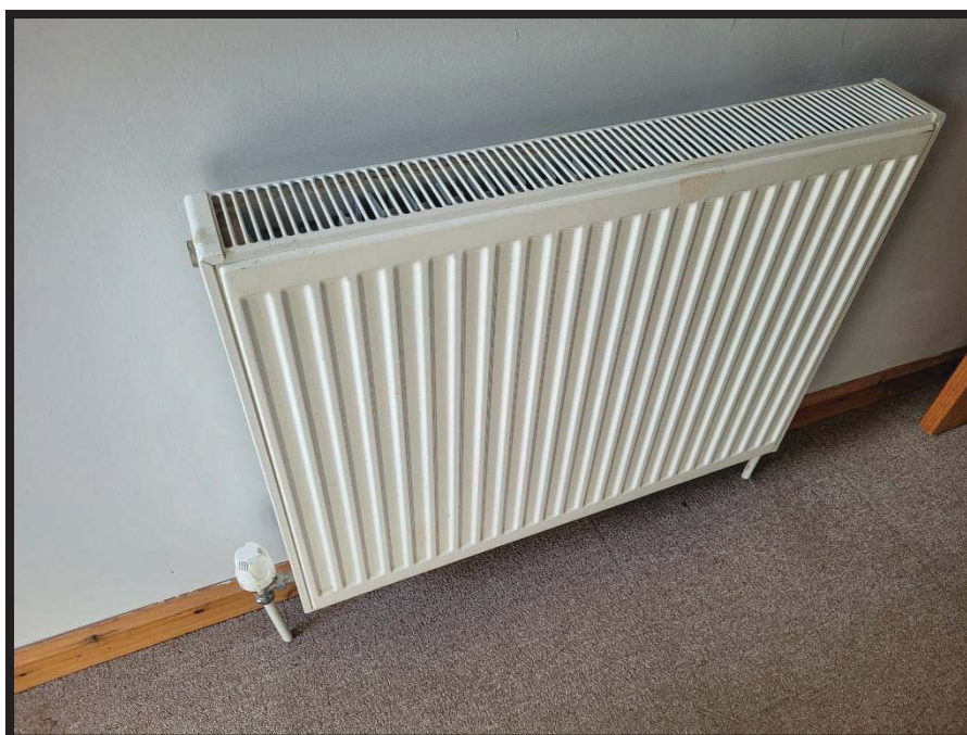
Photograph 8 Kitchen: Typical radiator with operational TRV.
