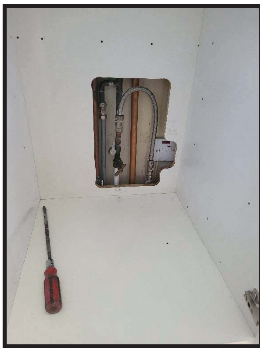
Photograph 11 Utility area: Internal water stop tap.
