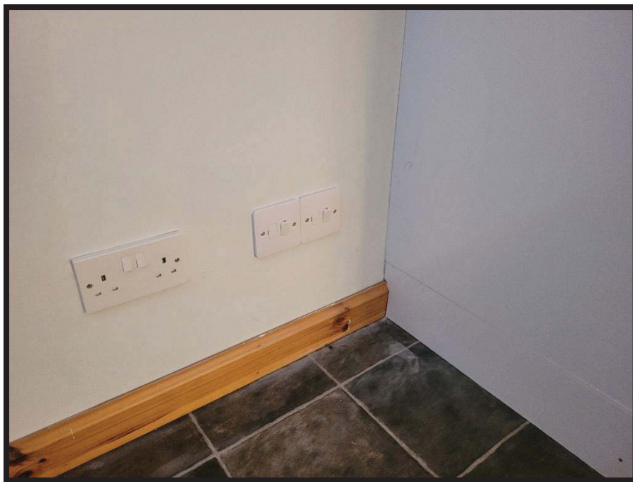
Photograph 9 Kitchen: Isolation switches for fridge/freezer.
