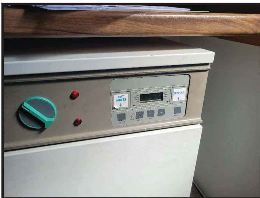
Photograph 10 Utility area: Boiler with integral programmer.
