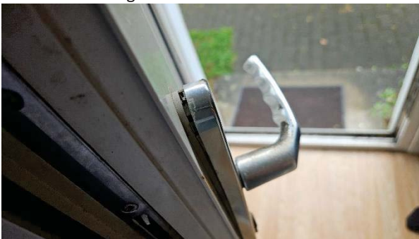
13 Lever handle to entrance door – cover plate loose.
