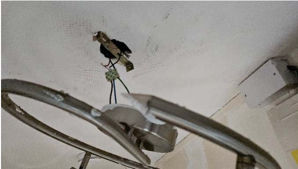
11 Hallway light fitting – hanging loose and not secured to ceiling bracket.
