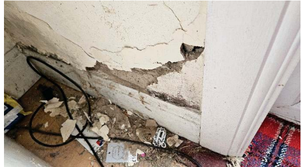
20 Defective plasterwork adjacent to rear door.
