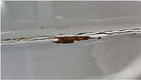
17 Minor water damage to bath panel.
