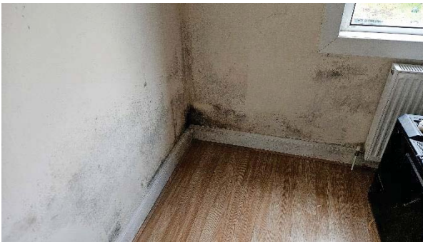
35 Bedroom – mould contamination.
