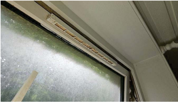
25 Trickle vent in closed position.
