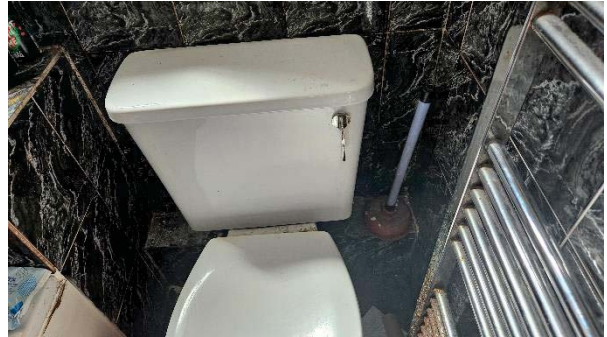
12 Defective cistern flush.
