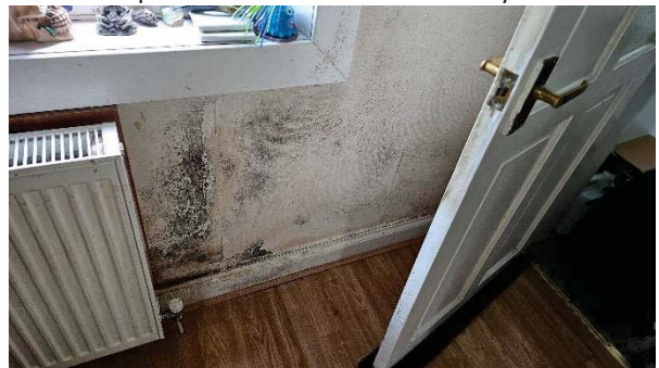
30 Living Room – mould present to external wall.
