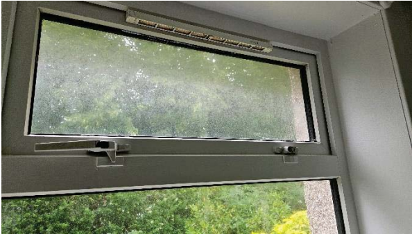
3 Damaged handle to kitchen window.
