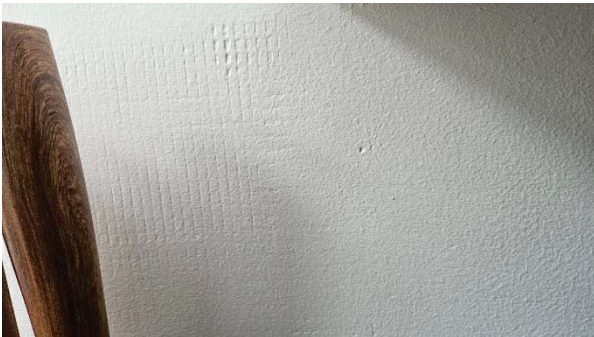
5 Example of incomplete filler over reinforcement tape to recent plastering works.
