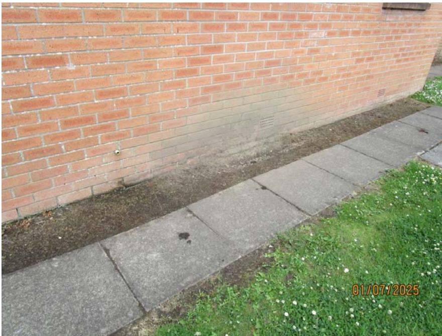
9. Staining at leaking gutter
