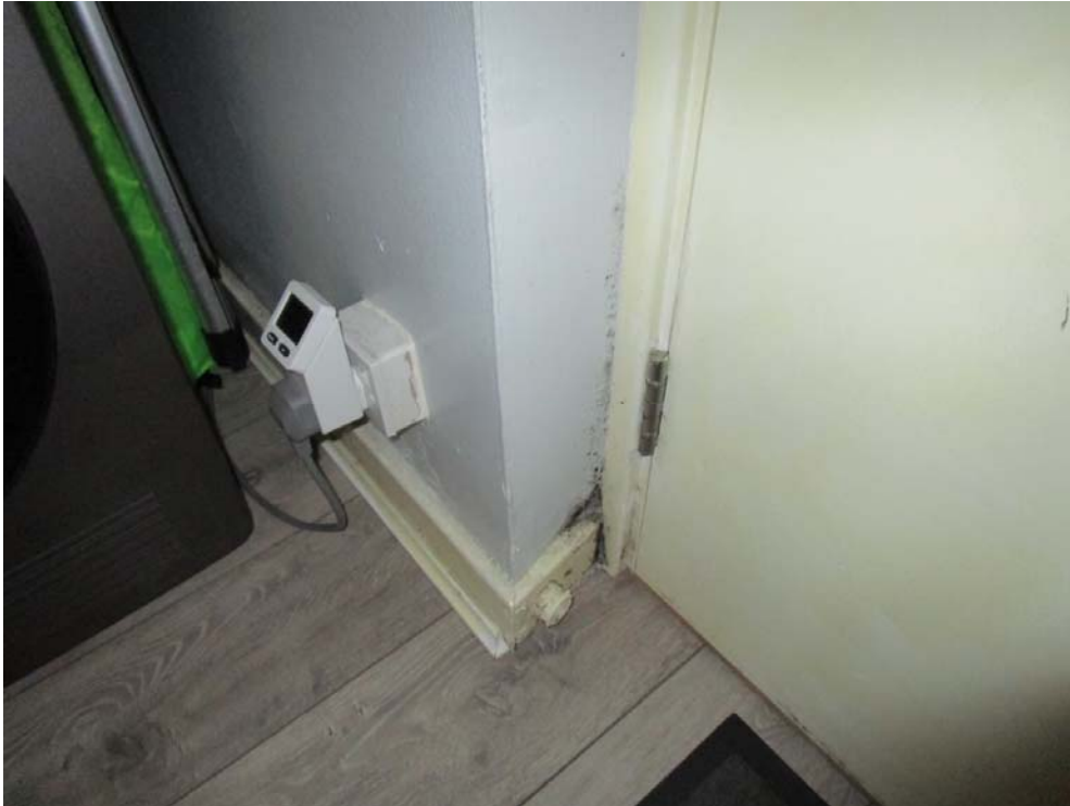
1. Mould and dampness adjacent front door
