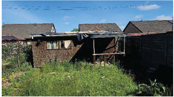
28 Dilapidated outbuilding with roof damaged.
