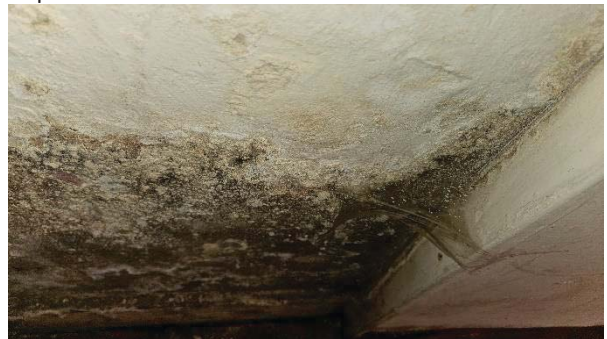
12 Blistering and deterioration of paint finish due to dampness.
