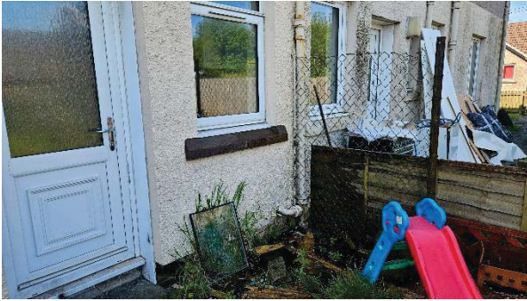
27 Overflow at eaves saturating base of wall and fence over rear elevation.
