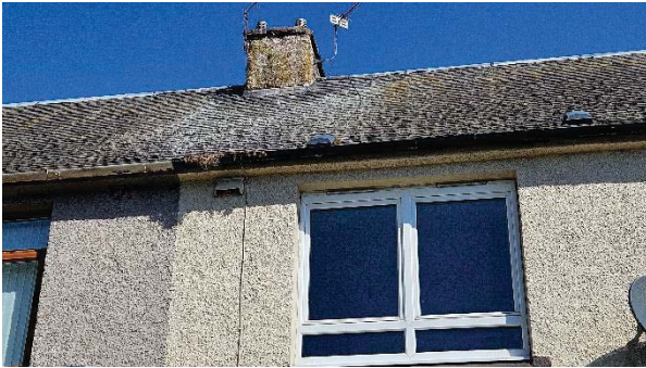
1 Visual vegetation evident to rainwater gutters at front roof pitch.
