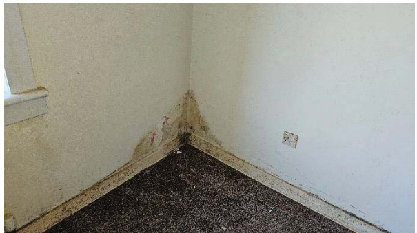
20 Rear Bedroom – dampness at corner to low level.
