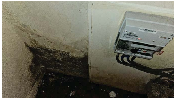
10 Heavy mould growth to external wall within Hall Cupboard.
