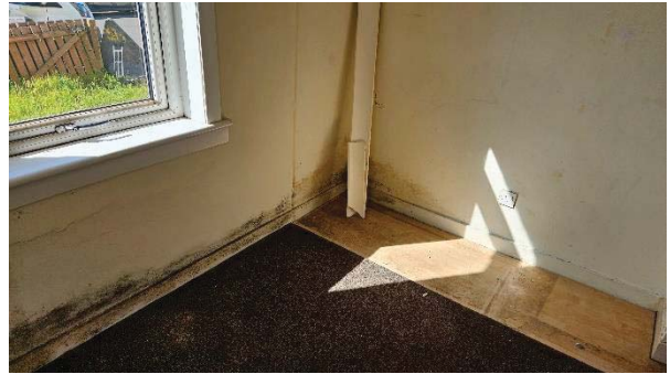
4 Visual mould growth evident at low levels to external walls within Eastmost Bedroom.
