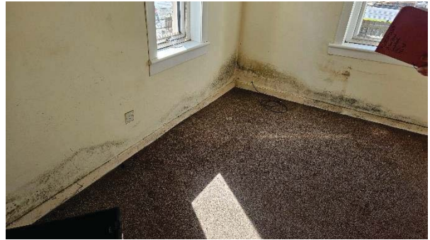
2 Visual mould growth evident at low levels to external walls within Eastmost Bedroom.
