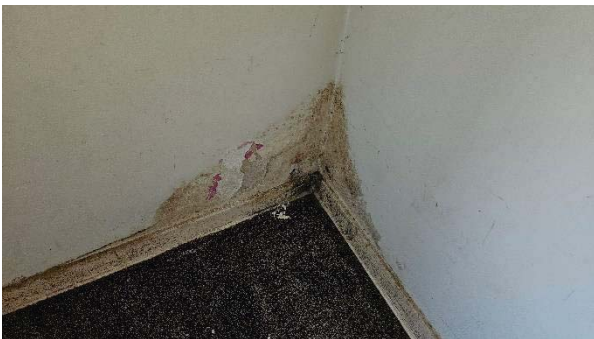
21 Rear Bedroom – dampness at corner to low level.
