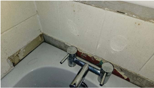
25 Missing tiles at junction with bath and not sealed.
