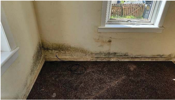
3 Visual mould growth evident at low levels to external walls within Eastmost Bedroom.
