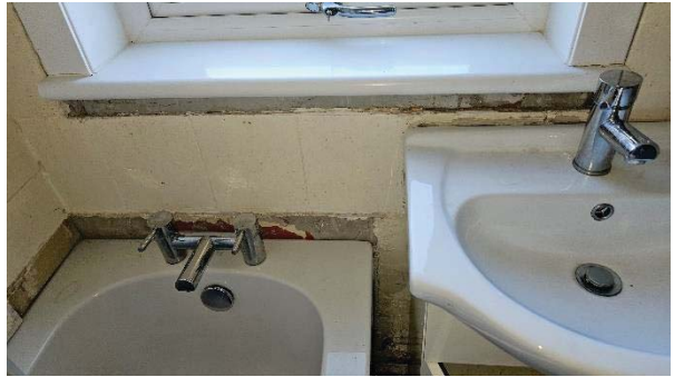
26 Missing tiles at junction with bath and not sealed.
