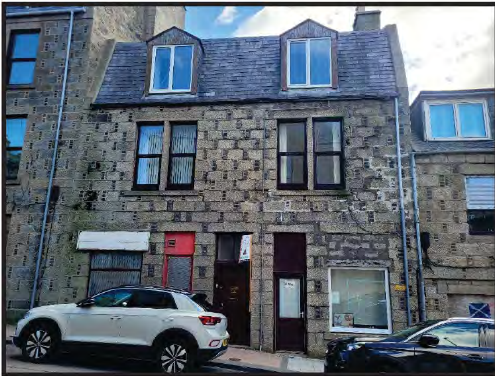
Photograph 1 Front (Western) Elevation. Vegetation at left side of gutter, gutter lined with "flashband", patch repairs to pointing right hand side front wall. Front windows replaced to first floor.
