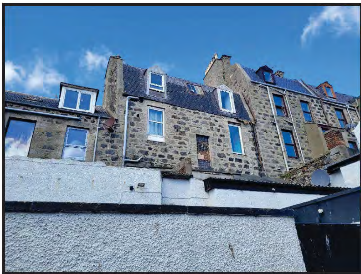
Photograph 4 Rear elevation: Appears unchanged. Gutter missing. Missing slates and deterioration of rear dormer window. Deterioration of skylight and stairwell window.
