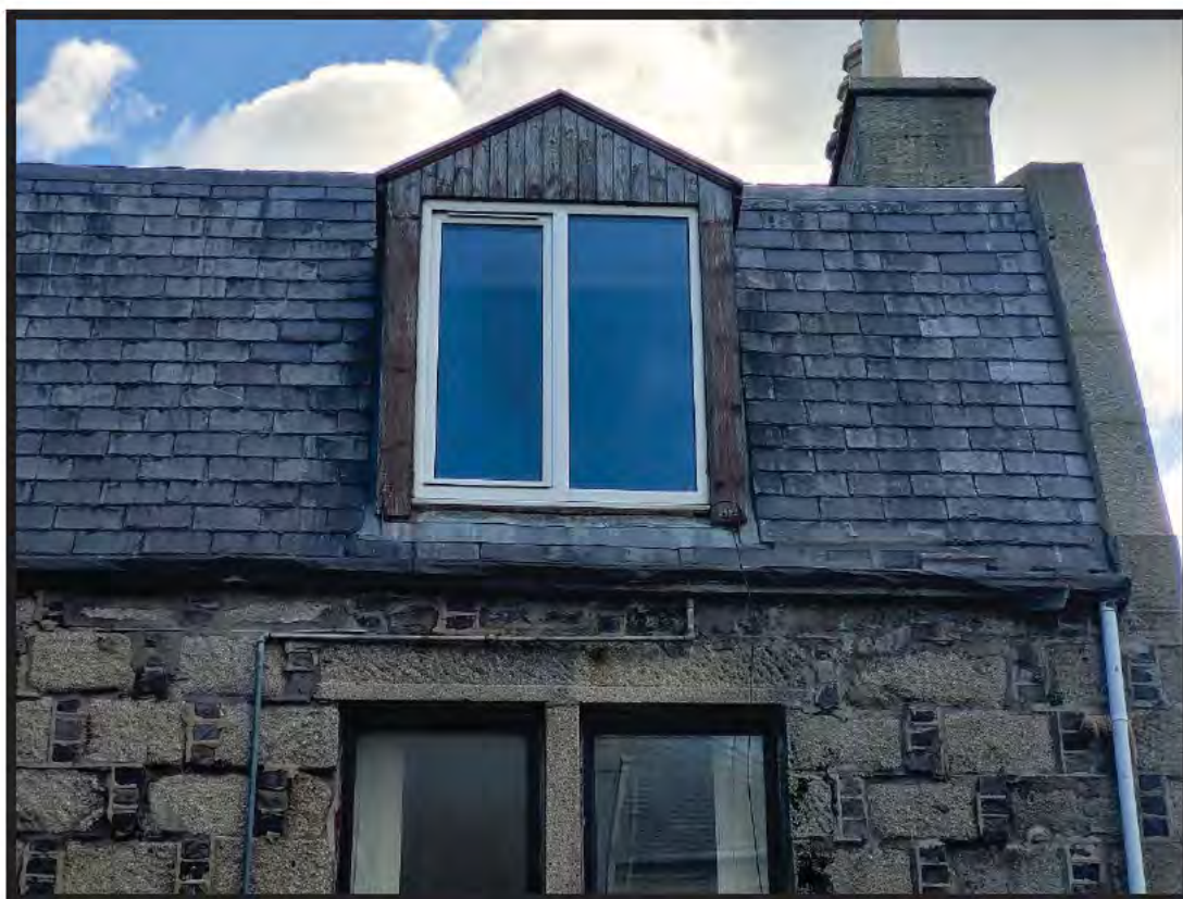
Photograph 2 Front elevation: Flashband applied to slates, right hand side of dormer
