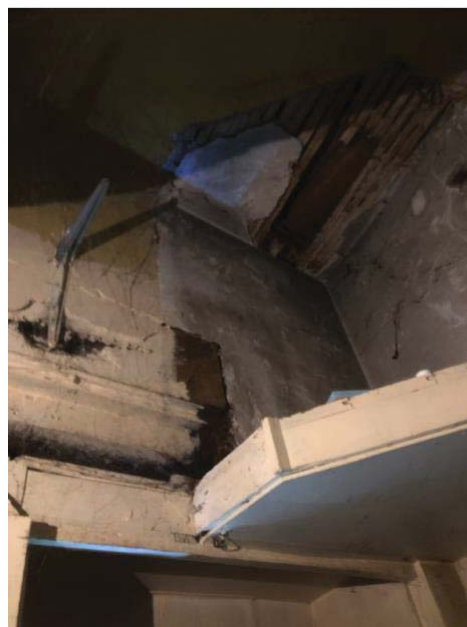
Photo 17 – Exposed lath and plaster in cup/b
