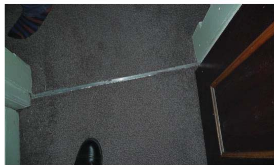
Photo 5 – Carpet not fixed under threshold plate
