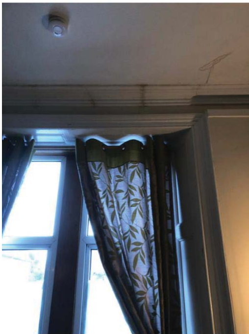
Photo 24 – Historic water ingress staining
