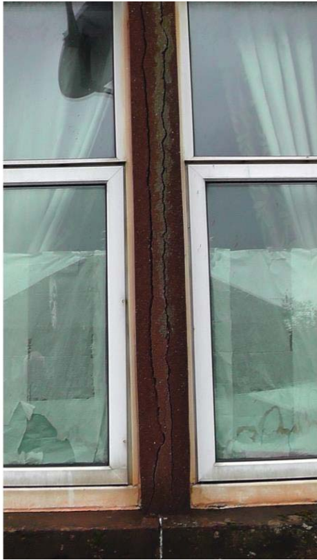
Photo 32 – Failing stone mullion
