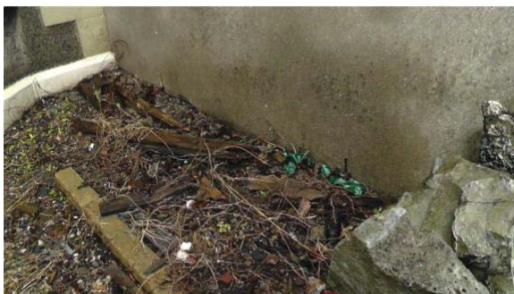
Photo 30 – Raised ground level + damp bridge
