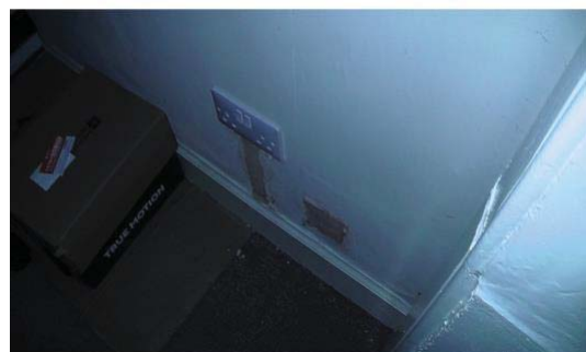
Photo 9 – Socket re-installation in Hallway
