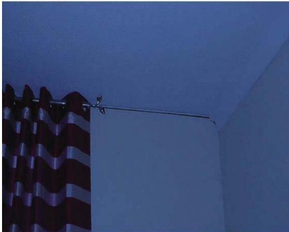
Photo 12 –Missing coving and gap in Bedroom wall
