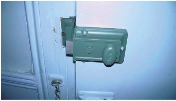
Photo 2 – Poorly secured and ill-fitting door
