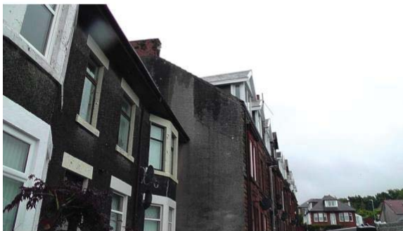
Photo 28 – Water staining on gable wall
