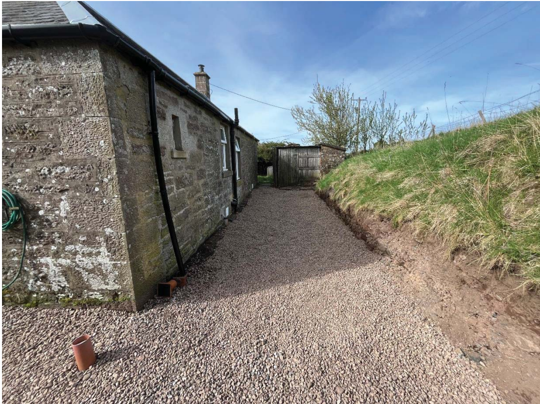
North elevation and garden excavated and reinstated where drainage installed.
