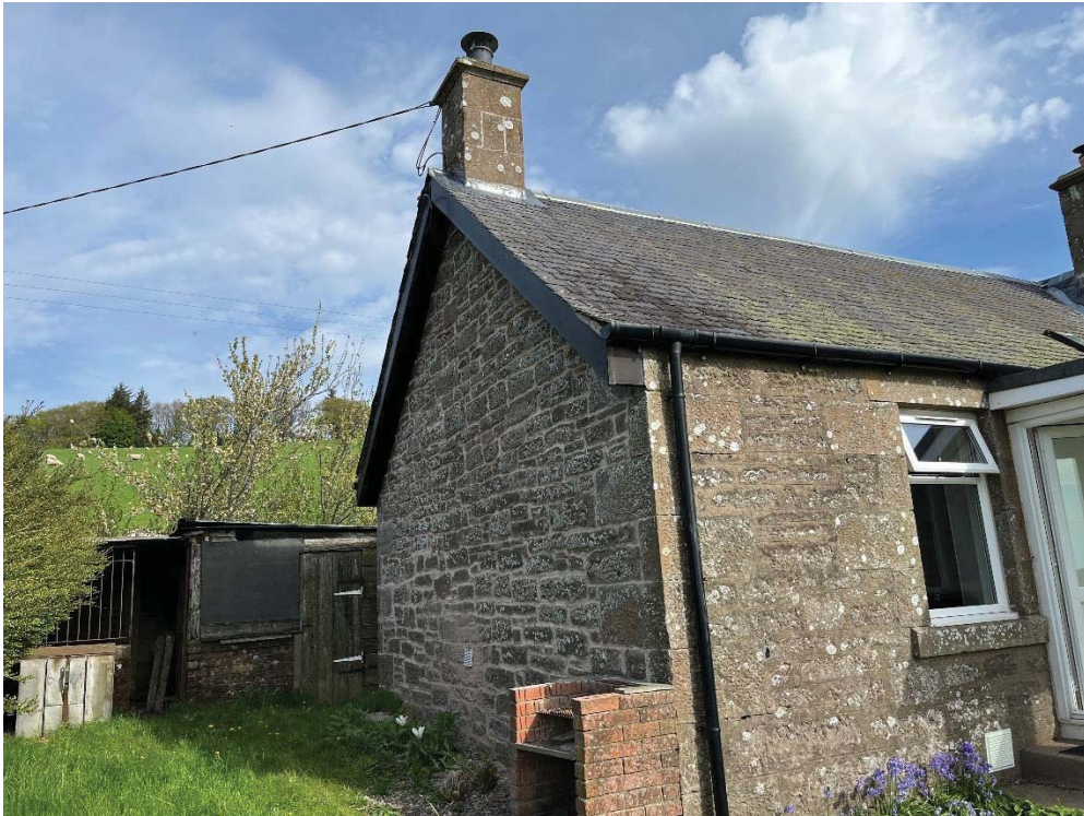
Repointed west gable wall. Vegetation removed.
