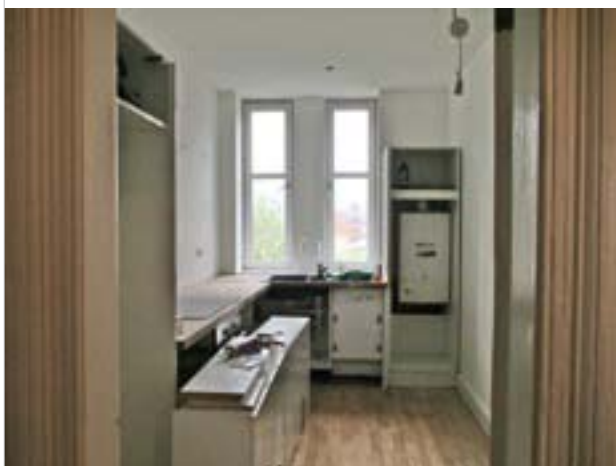
Kitchen - wall mounted units and base unit doors removed during renovation work (observation)
