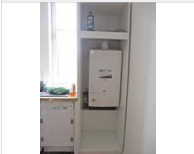
Kitchen - boiler - door of cupboard housing appliance removed and no CO alarm (observation)
