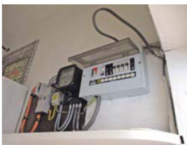
Hall Cupboard - wall mounted electrical consumer unit
