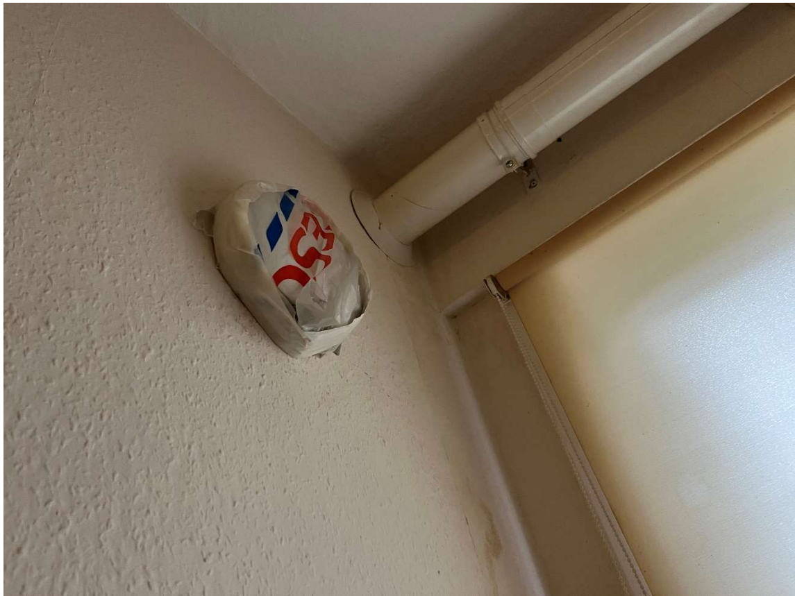
Vent in Kitchen covered with plastic bag.
