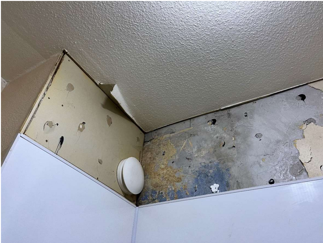
Damaged wall finish and decoration in Shower Room.
