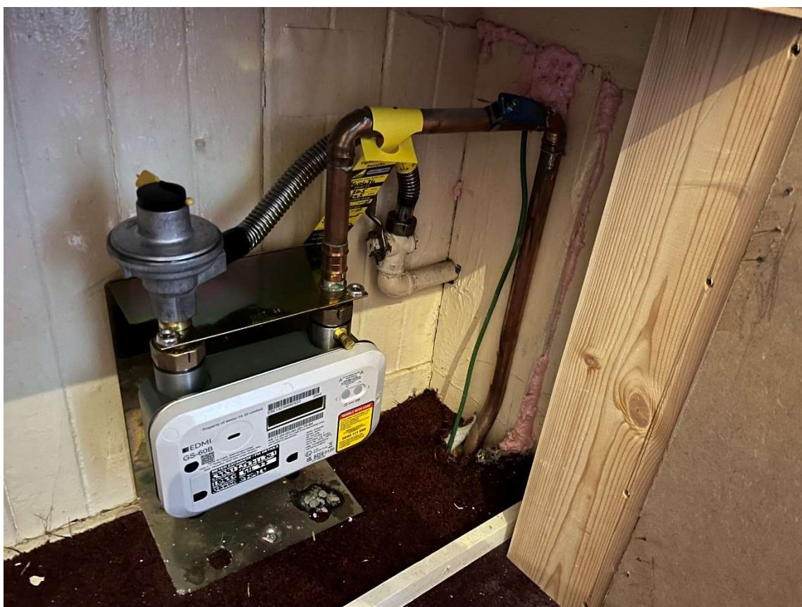
Gaps in lining boards of gas meter cupboard sealed with expanded foam.
