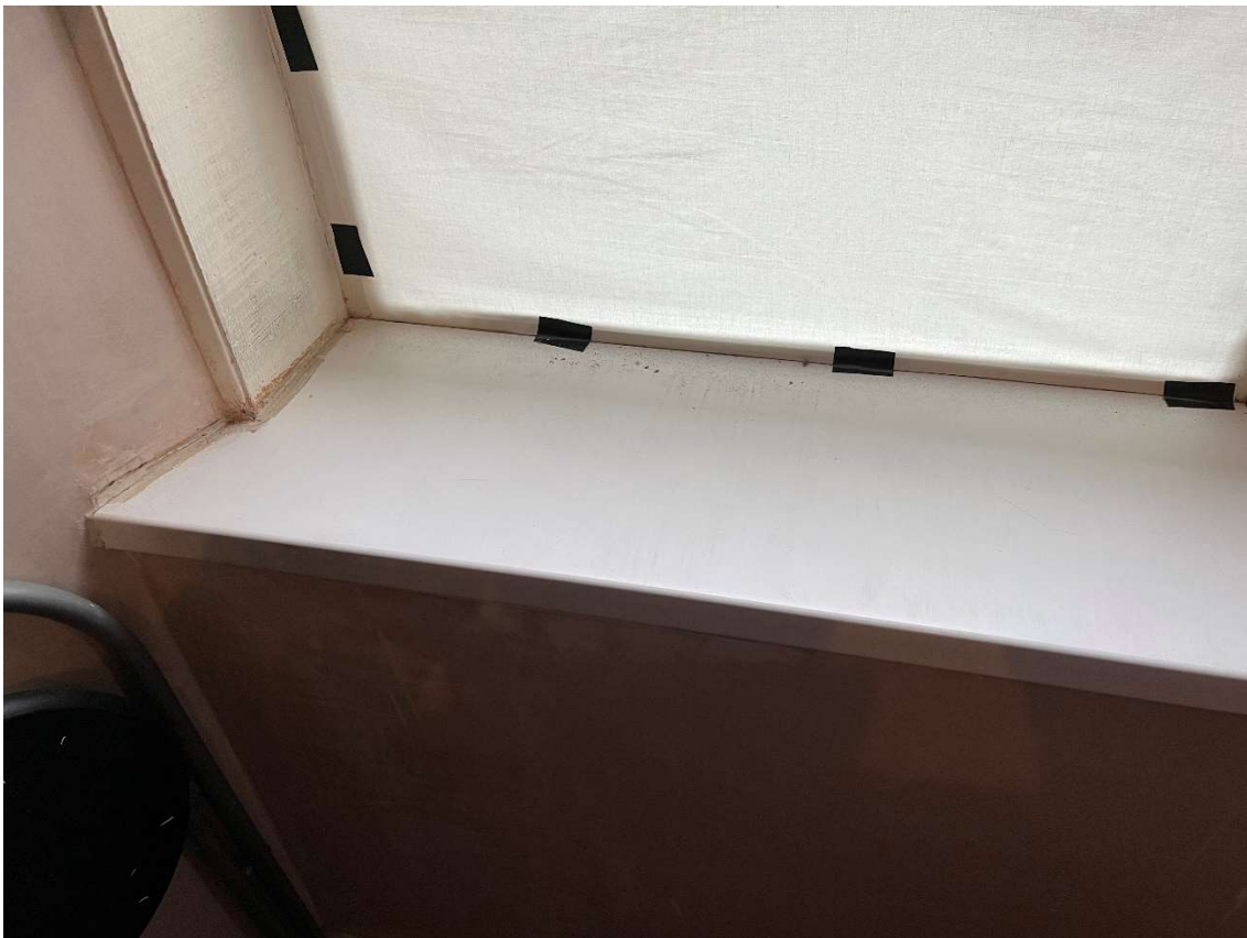
Loose/poorly sealed window sill in Front Room.
