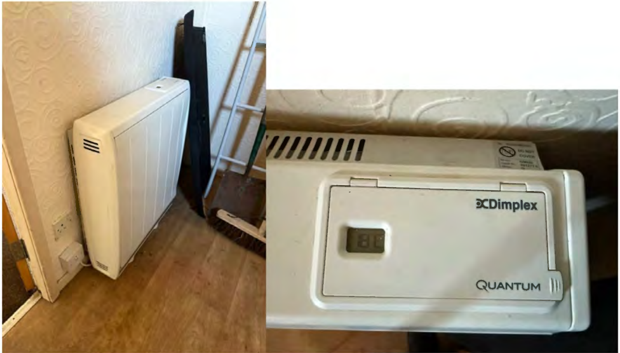
Photograph 2 and 3: Downstairs hallway: Electric storage heater
