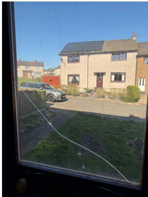
Photograph 6: Living room: Front window cracked
