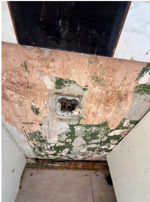
Photograph 14: Kitchen: Cooker space – bare wires
