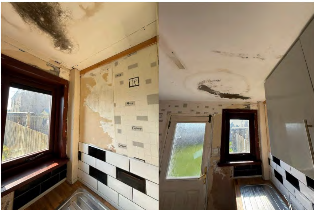
Photographs 15 and 16: Kitchen: Leak from bathroom and peeling wallpaper
