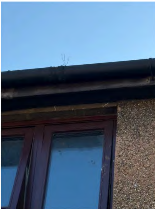
Photographs 39 and 40: Front elevation: Vegetation to guttering
