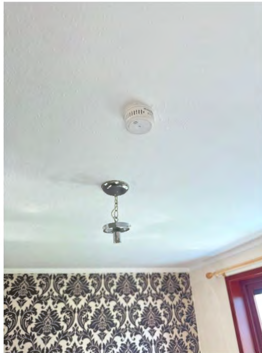
Photograph 7: Living room: Smoke detector (not interlinked)
