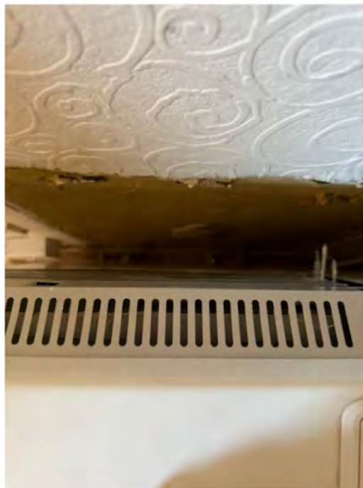
Photograph 4: Downstairs hallway: Electric storage heater not attached to wall
