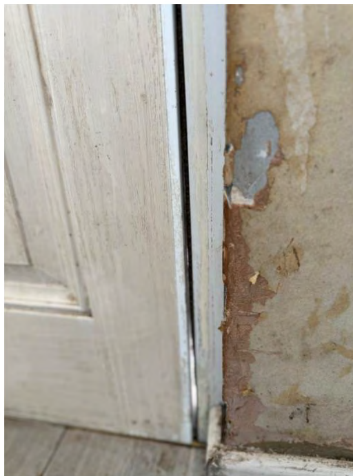
Photograph 18: Kitchen: Ill-fitting back door
