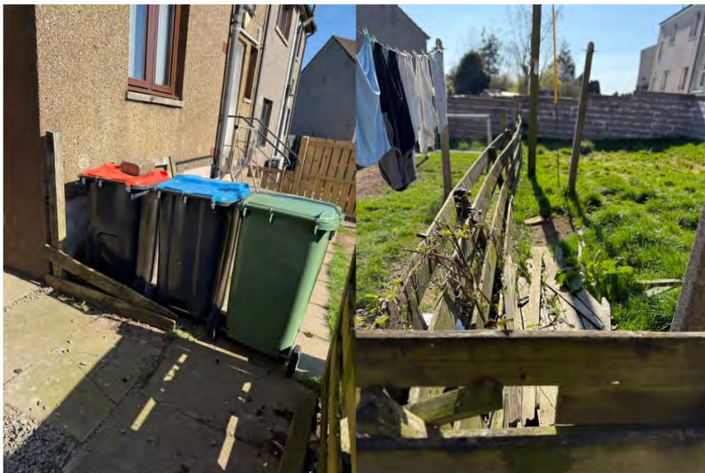
Photographs 36 and 37: Rear elevation: Fence and gate broken
