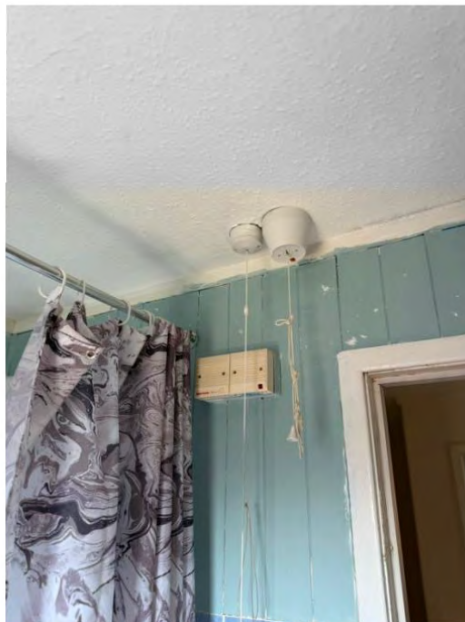
Photograph 20: Bathroom: Light switch and shower switch (light not working)
