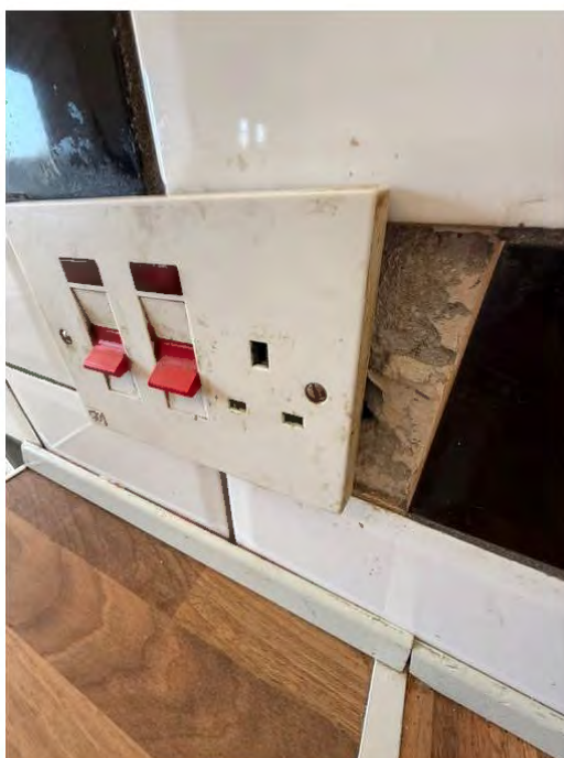
Photograph 13: Kitchen: Cooker isolator/plug – not fixed to wall
