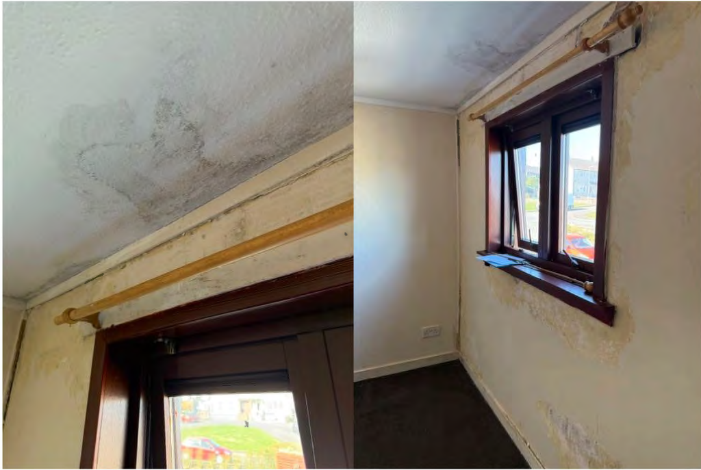
Photograph 30: Bedroom 2 (rear): Mould to ceiling; window and curtain pole fascia
