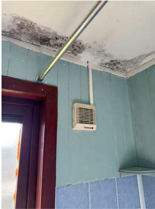
Photograph 23: Bathroom: Mould to ceiling and extractor unit
