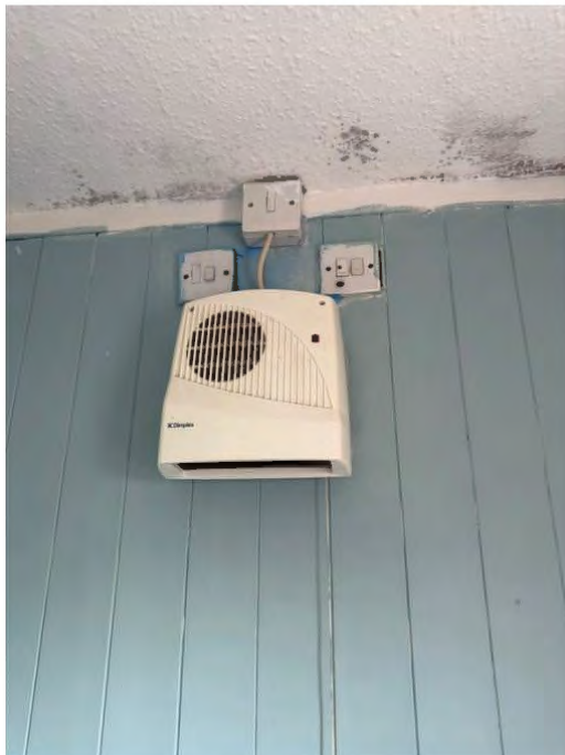
Photograph 22: Bathroom: Mould to ceiling and heater
