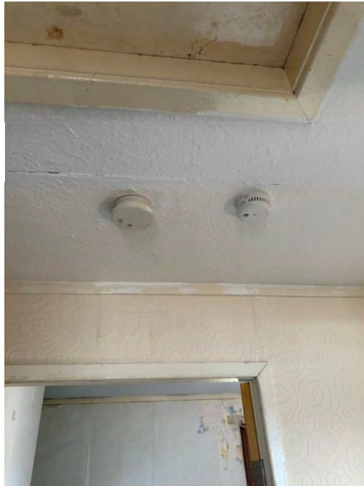
Photograph 19: Upstairs landing: Smoke detectors (not interlinked)
