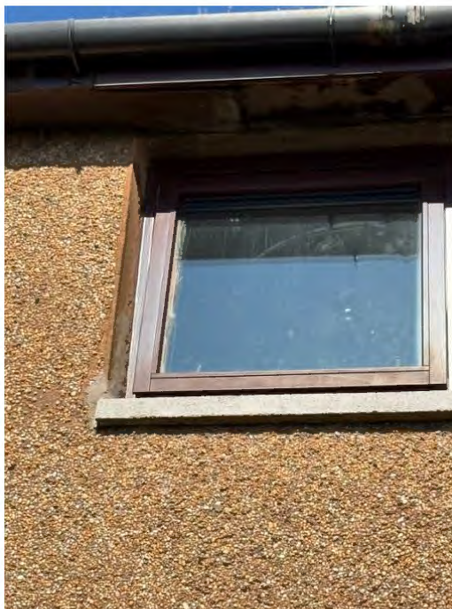
Photograph 34: Rear elevation: Soffit board not secured
