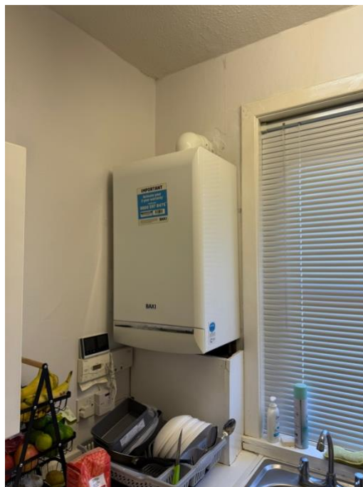
Photograph 5: Kitchen: Gas boiler
