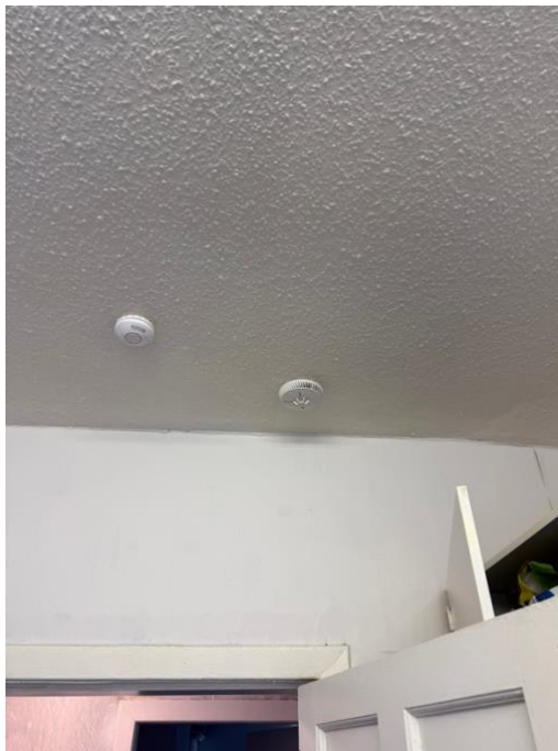
Photograph 3: Kitchen: smoke and heat detectors (latter is interlinked)
