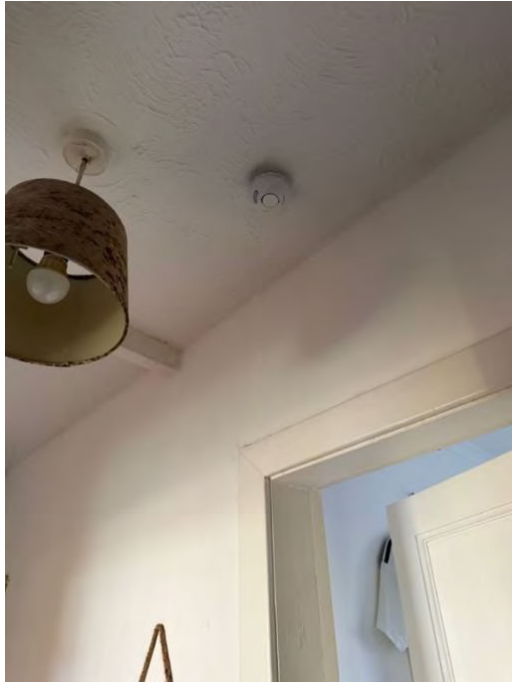
Photograph 9: Living room: Smoke detector
