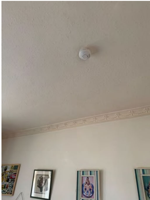
Photograph 9: Living room: Smoke detector
