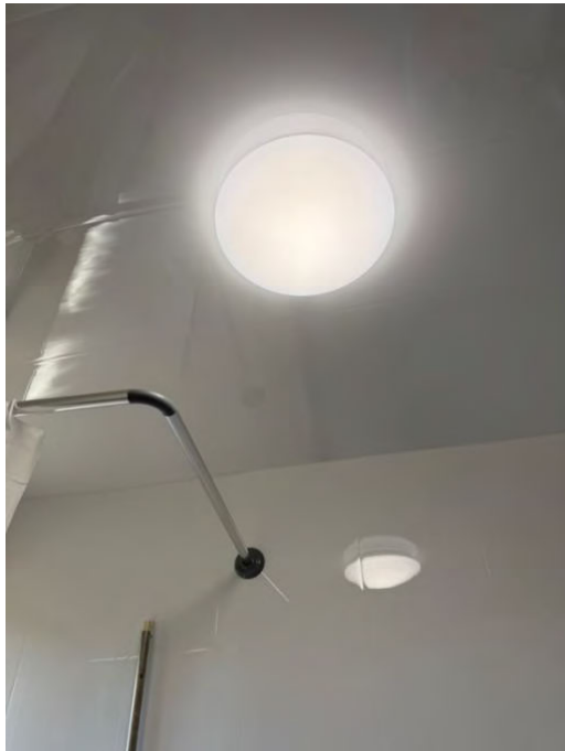
Photograph 13: Bathroom: ceiling light
