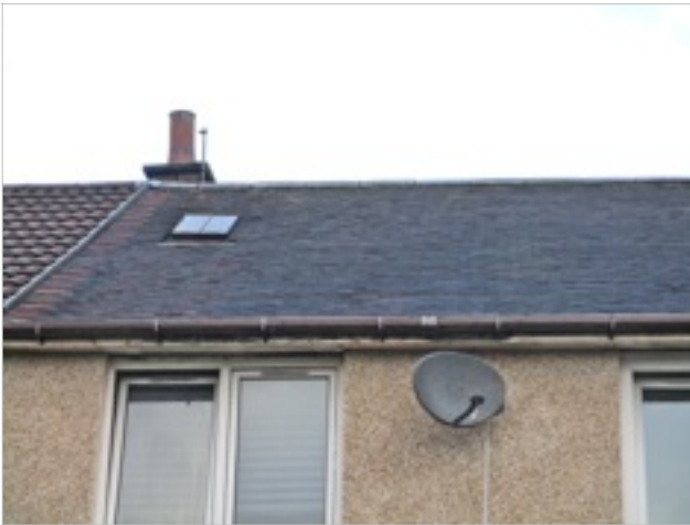
Rear elevation showing roof
