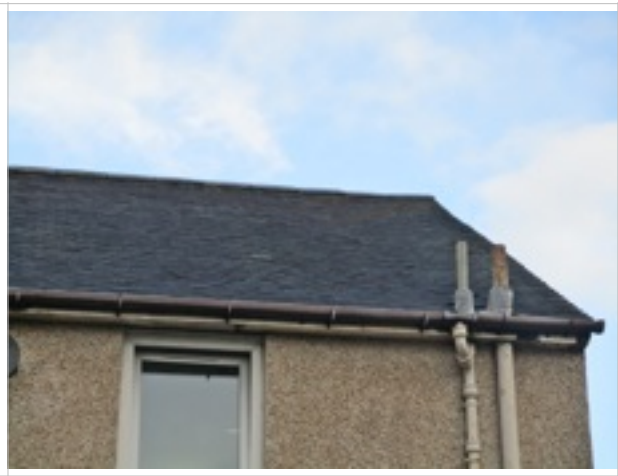
Rear elevation showing roof
