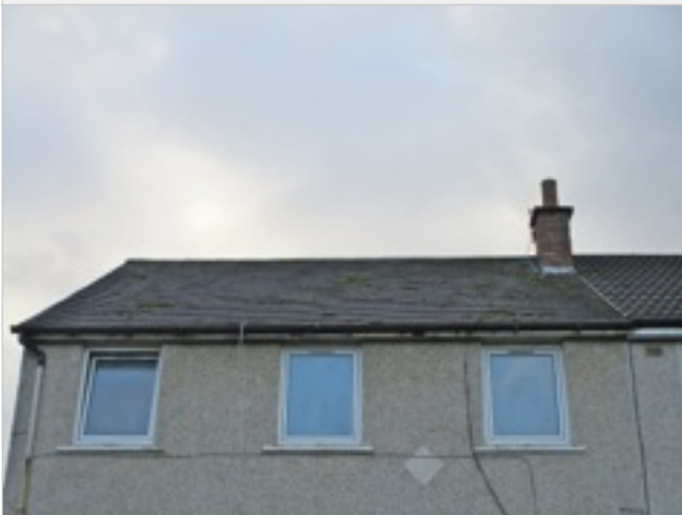
Front elevation showing roof
