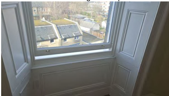
5 Internal view of new Rear Bedroom window.
