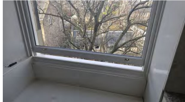
4 Internal view of new Kitchen window.
