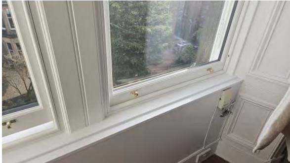
3 Internal view of new Living Room bipartite window.
