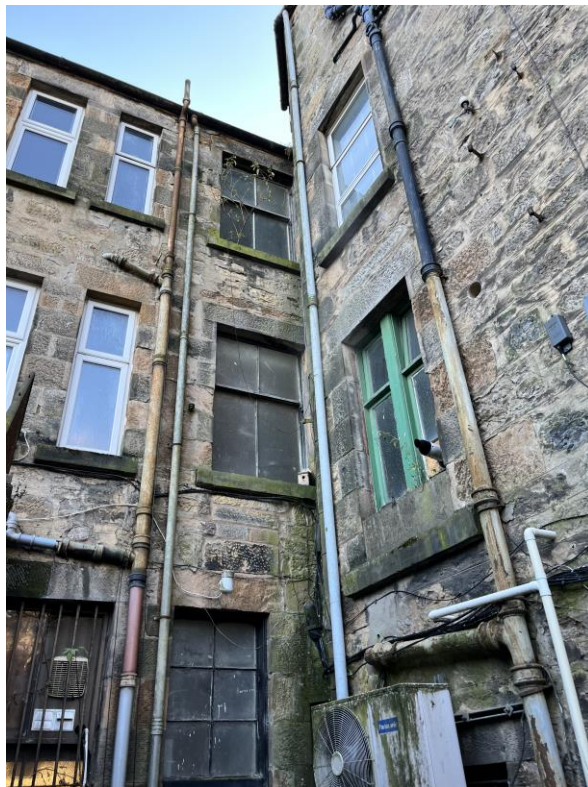
Rear of the building
