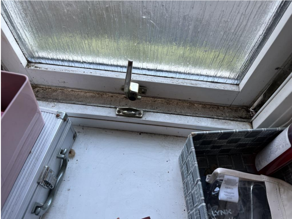
Draughtproofing strip evident
