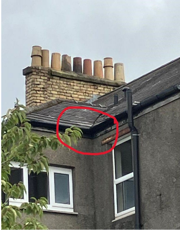
24 August 2024 - Roof & Valley gutter
