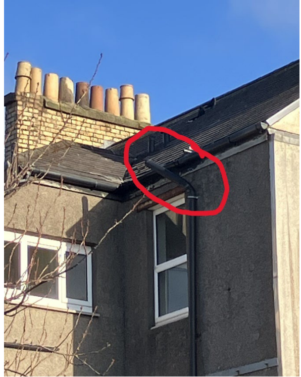
10 February 2025- Roof & Valley Gutter
