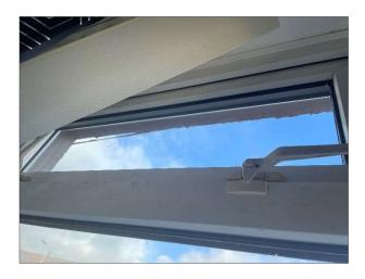
Seal around window has failed and a gap is noticeable between the double-glazed unit and the window frame. A draught was noted during the inspection.
