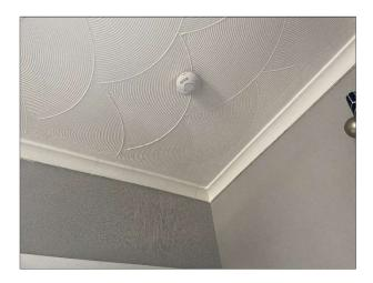
A smoke detector was fitted in the lounge, ground and first floor hall and a heat detector was fitted in the kitchen. Each detector was tested and worked independently; however, no detector was interlinked.
