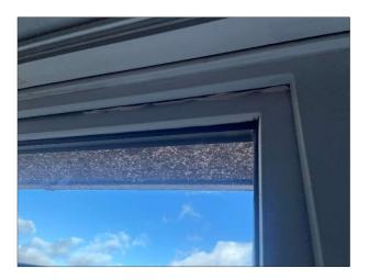
Seal around window has failed and a gap is noticeable between the double-glazed unit and the window frame. A draught was noted during the inspection.
