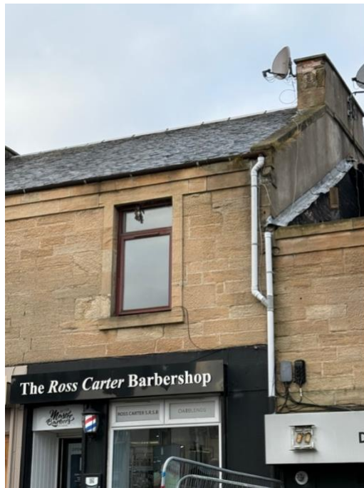
Photograph 2: Front right-hand corner of roof
