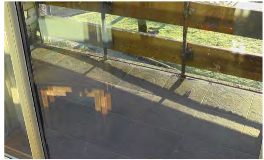
Photo 3 – Replaced Balcony surface
