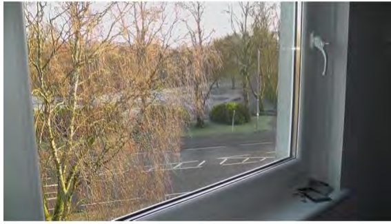
Photo 10 – New window unit in Bedroom 2
