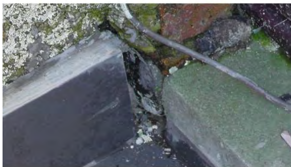
Photo 6 – Unfinished upstand detail at Balcony door
