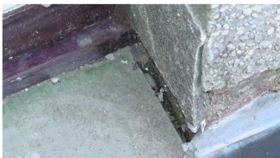
Photo 6 – Unfinished upstand detail at Balcony door
