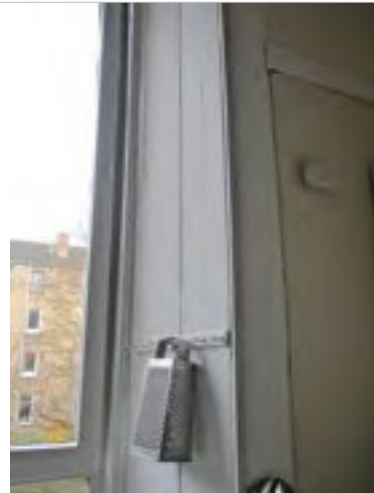
Kitchen - timber panelling to right side of window
