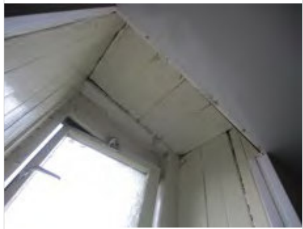
Bathroom - timber panelling above and around window
