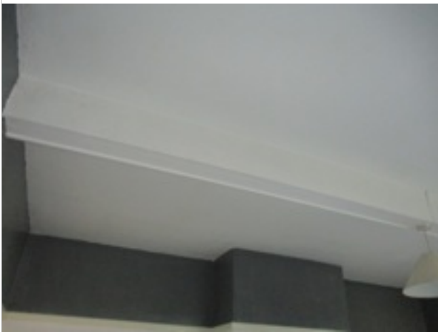
Front Bedroom - ceiling
