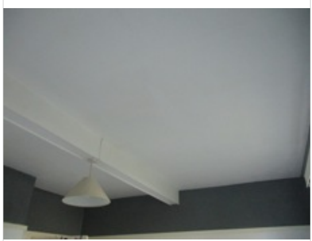
Front Bedroom - ceiling
