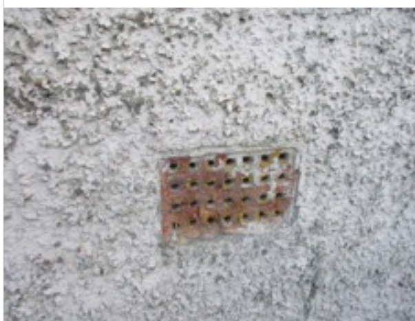
Front Elevation - underfloor vent - cleared and situated well above ground level
