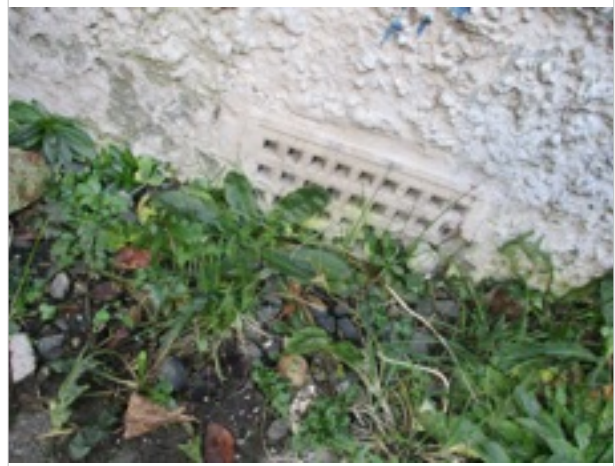
Rear Elevation - underfloor vent part obscured by path/flower bed
