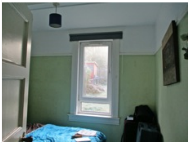
Rear Bedroom - rear external wall
