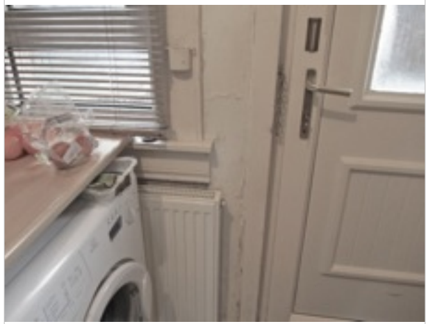
Kitchen - rear external wall
