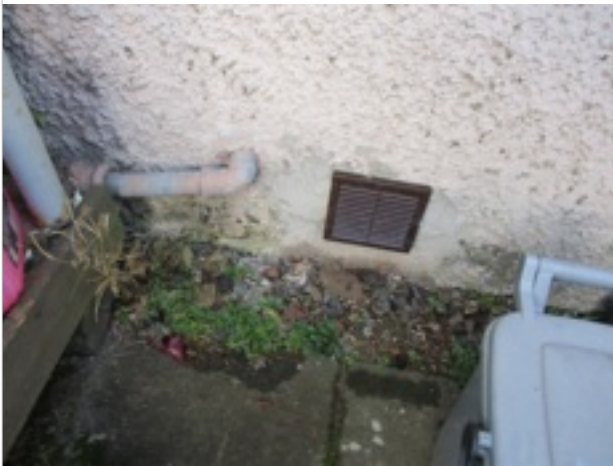
Rear Elevation - new underfloor vent cover
