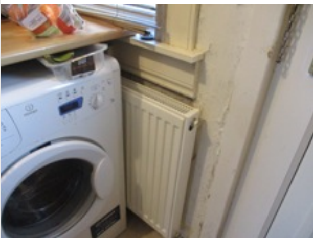
Kitchen - new radiator
