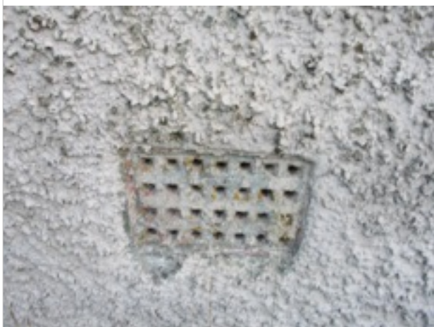
Front Elevation - underfloor vent - cleared and situated well above ground level
