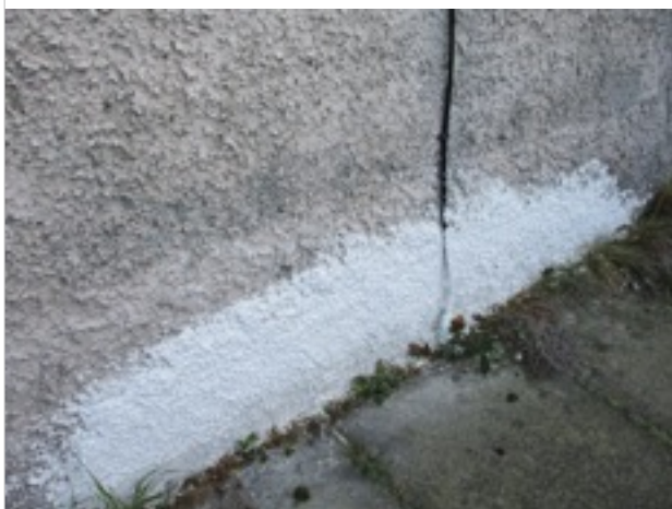
Front Elevation - roughcast patched
