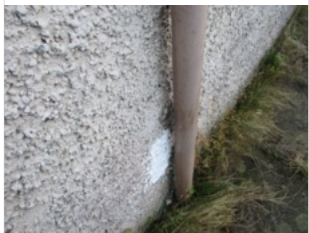
Front Elevation - roughcast patched
