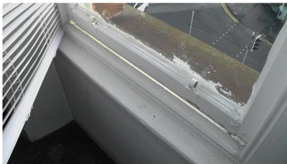
Photo 4 – Functioning sash window in Living Room
