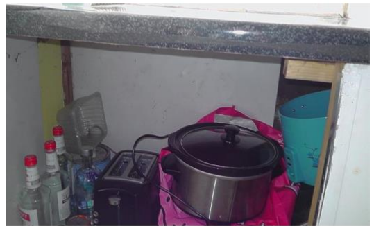
Photo 7 – No issue identified below Kitchen window
