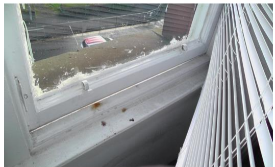
Photo 5 – Functioning sash window in Living room
