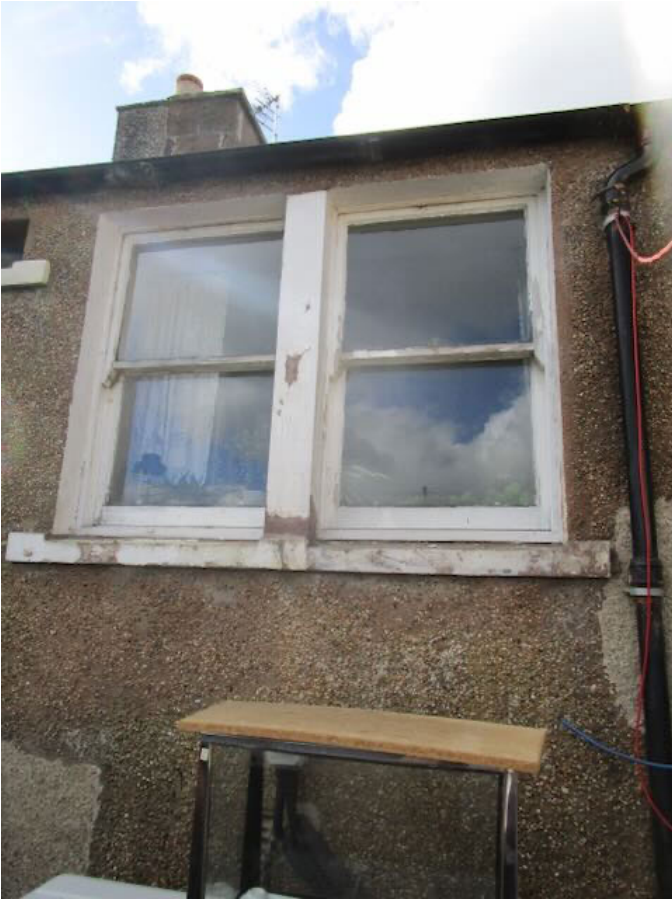
11. Window and gutters to rear
