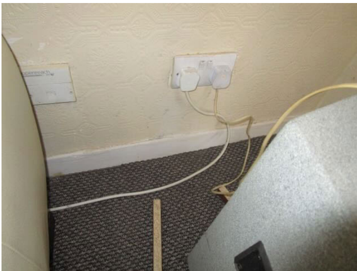
2. Damp patch in living room.
