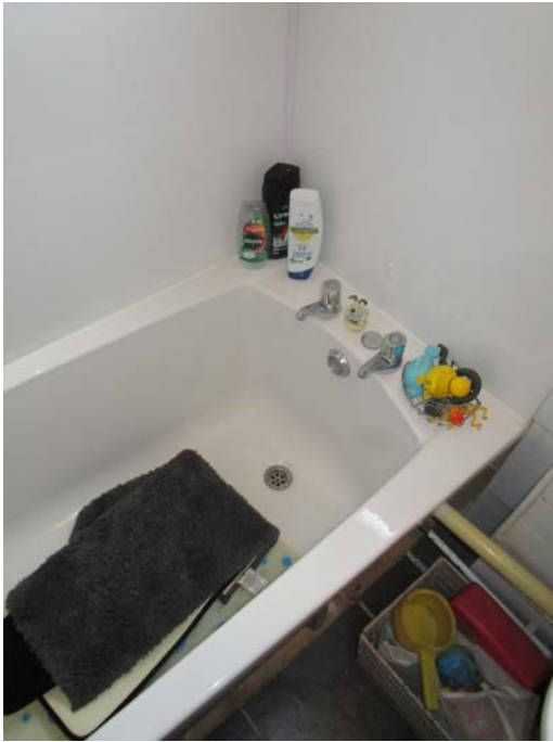
1. Bath, wetwall boarding and silicone seal.
