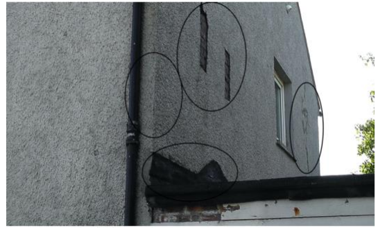
Photo 19 – Bossed roughcast/exposed brickwork
