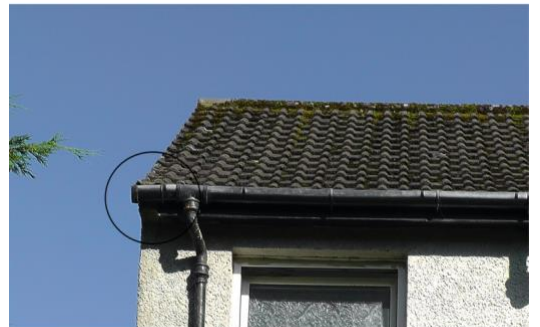
Photo 13 – Pitch/run issue with rear gutter
