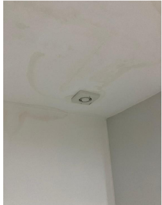
30 August 2024 – Bathroom vent
