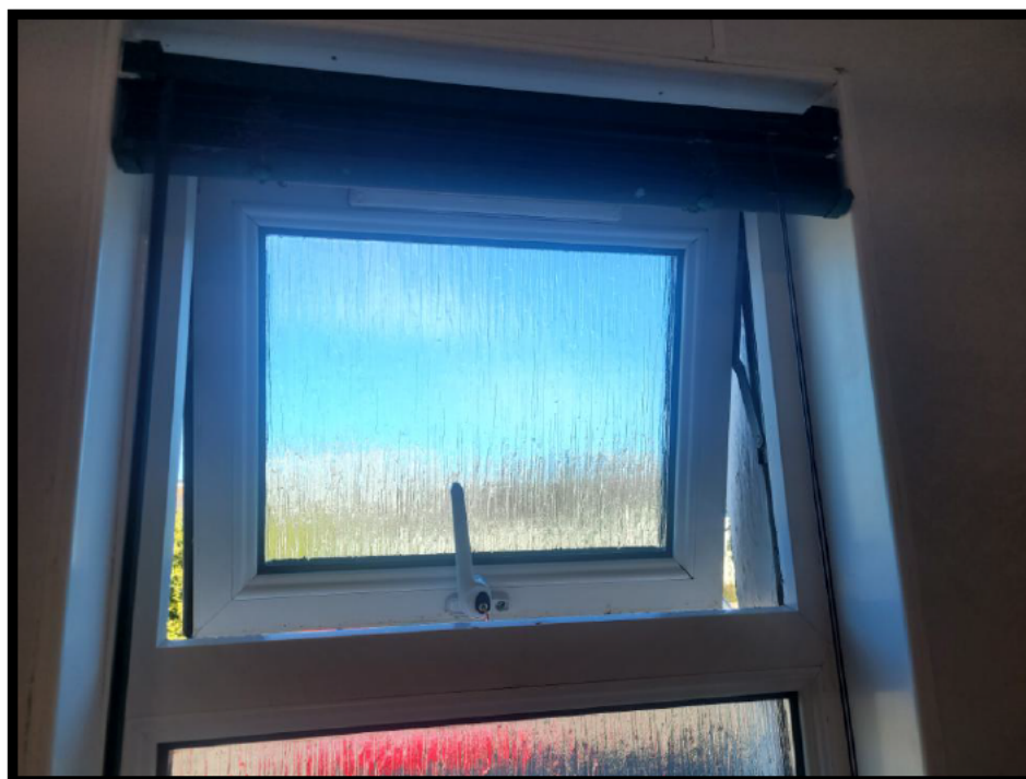
Photograph 4 Bathroom: Window opens and shuts as designed. Trickle vent present.
