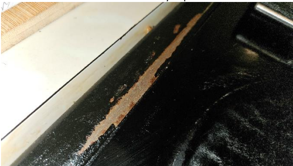
5 Example of localised area of defective coating to freestanding cooker.
