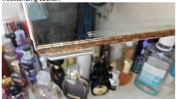
8 Bathroom cabinet – corrosion evident along metal retention trim.
