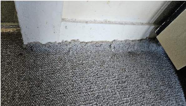
1 Perimeter of carpet floor covering at skirting junction.
