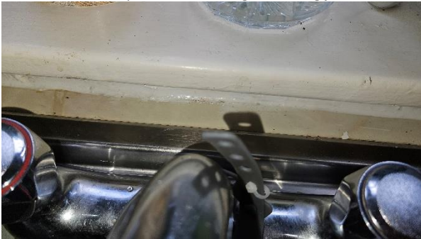
3 Silicon sealant in Kitchen recently replaced.
