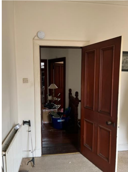
Photograph 9: Bedroom 3 – smoke detector just above door frame
