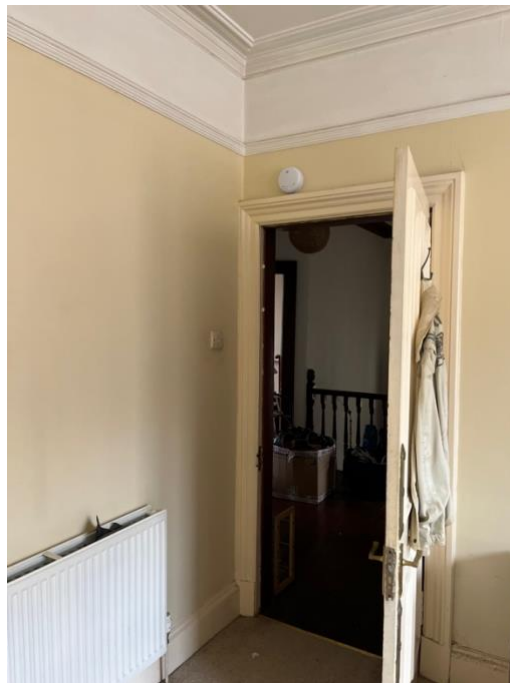
Photograph 9: Bedroom 3 – smoke detector just above door frame
