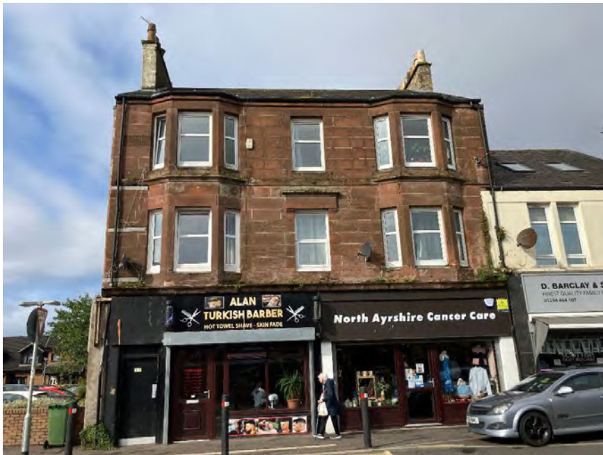
1. Front elevation as viewed from road.
