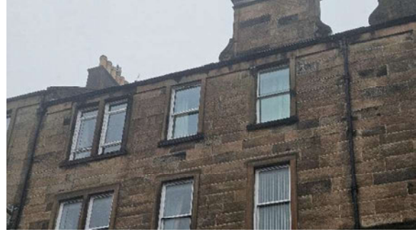
2 Third Floor flat windows viewed from street level.
