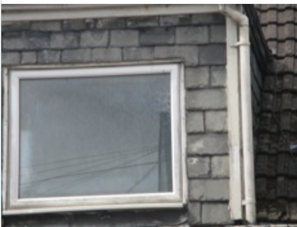
Rear Elevation - pvc gutter and downpipes to dormer window
