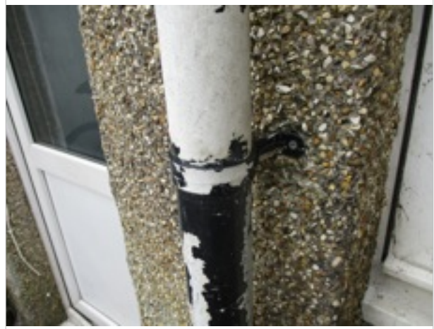
Rear Elevation - downpipe secured to wall
