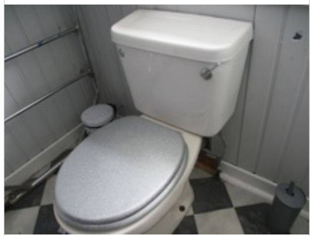
Bathroom - new pipe at toilet
