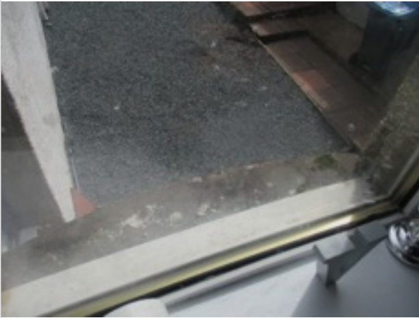
Hall/staircase - window sill internal and external view
