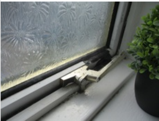
Bathroom - window - duct tape applied to base of frame
