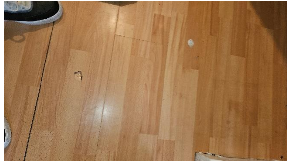
12 Example photograph of laminate flooring.
