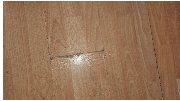
10 Example photograph of laminate flooring.
