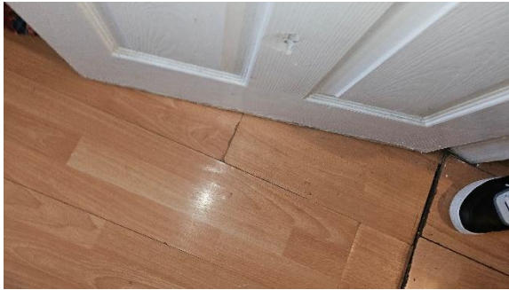
11 Example photograph of laminate flooring.
