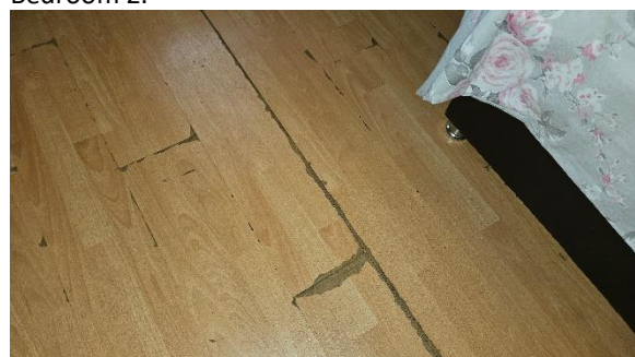
18 Example photograph of laminate flooring – Bedroom 2.
