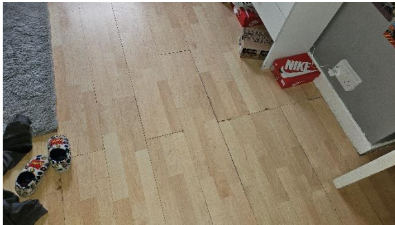
5 Example photograph of laminate flooring – Bedroom 1.
