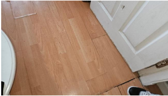
9 Example photograph of laminate flooring.
