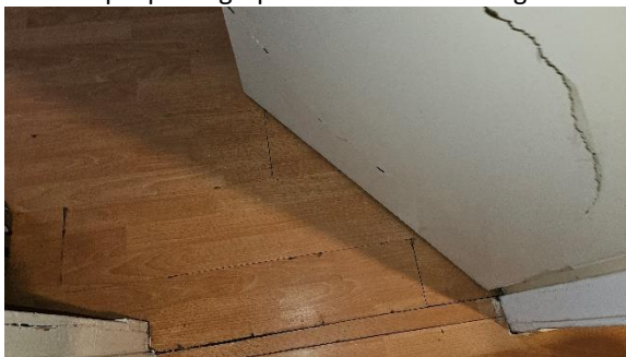
15 Example photograph of laminate flooring – Bedroom 2.
