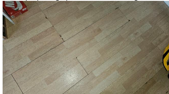
6 Example photograph of laminate flooring – Bedroom 1.
