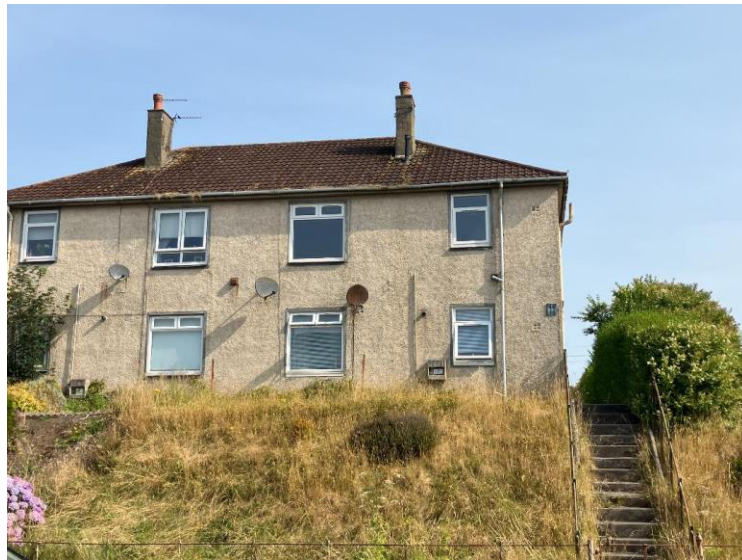
1. Front elevation as viewed from road.
