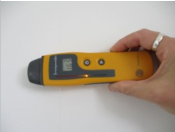
Front bedroom - internal party wall - damp meter reading showing moderate moisture level (search mode)
