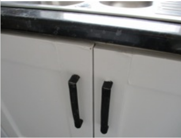
Kitchen - double base unit under sink - left side door does not close properly/misaligned
