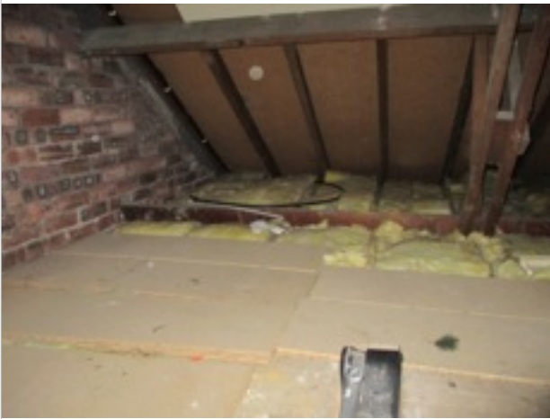
Loft - view towards rear pitch/gable wall/part floored
