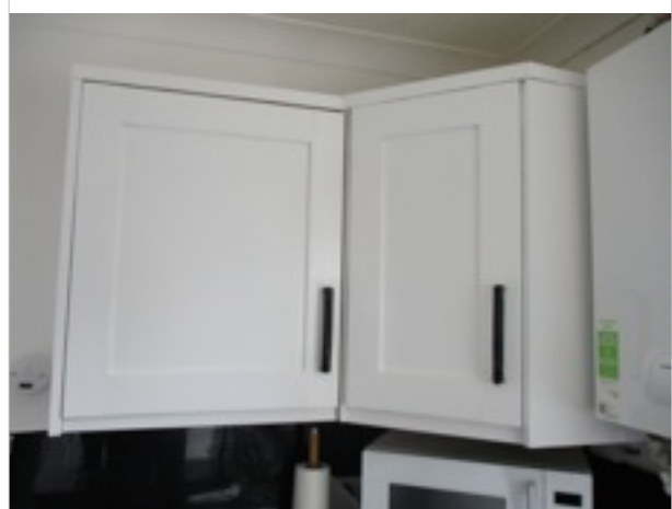
Kitchen - corner wall mounted units appear sound
