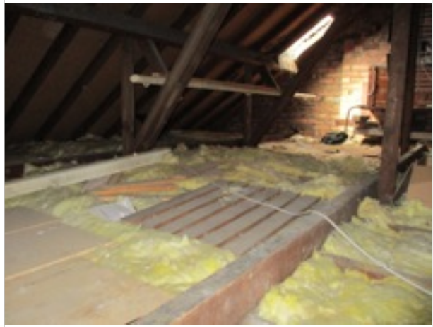
Loft - view towards party wall and skylight on rear pitch
