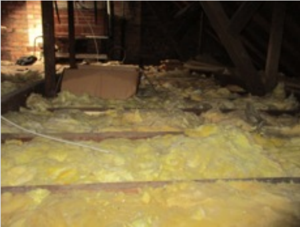
Loft - view towards party wall showing insulation
