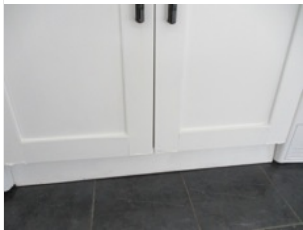
Kitchen - double base unit under sink - new kick board
